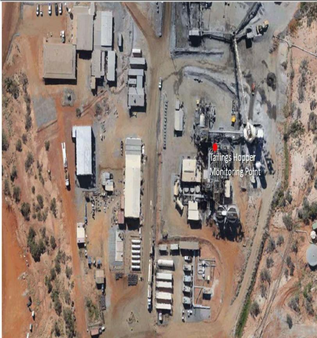
Figure 8: Tailings hopper monitoring point
