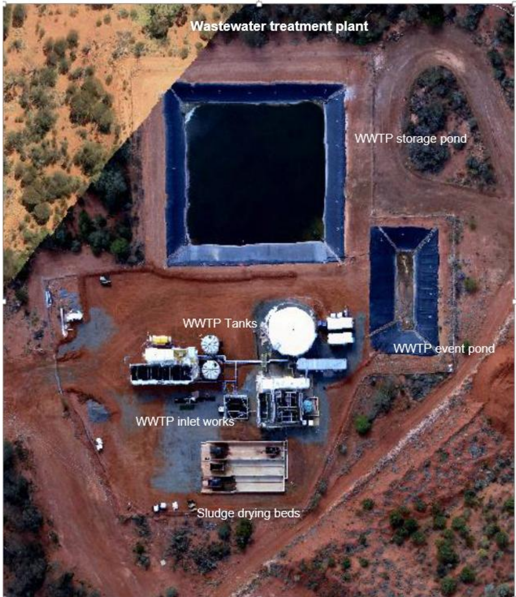
Figure 4: Wastewater treatment plant infrastructure
