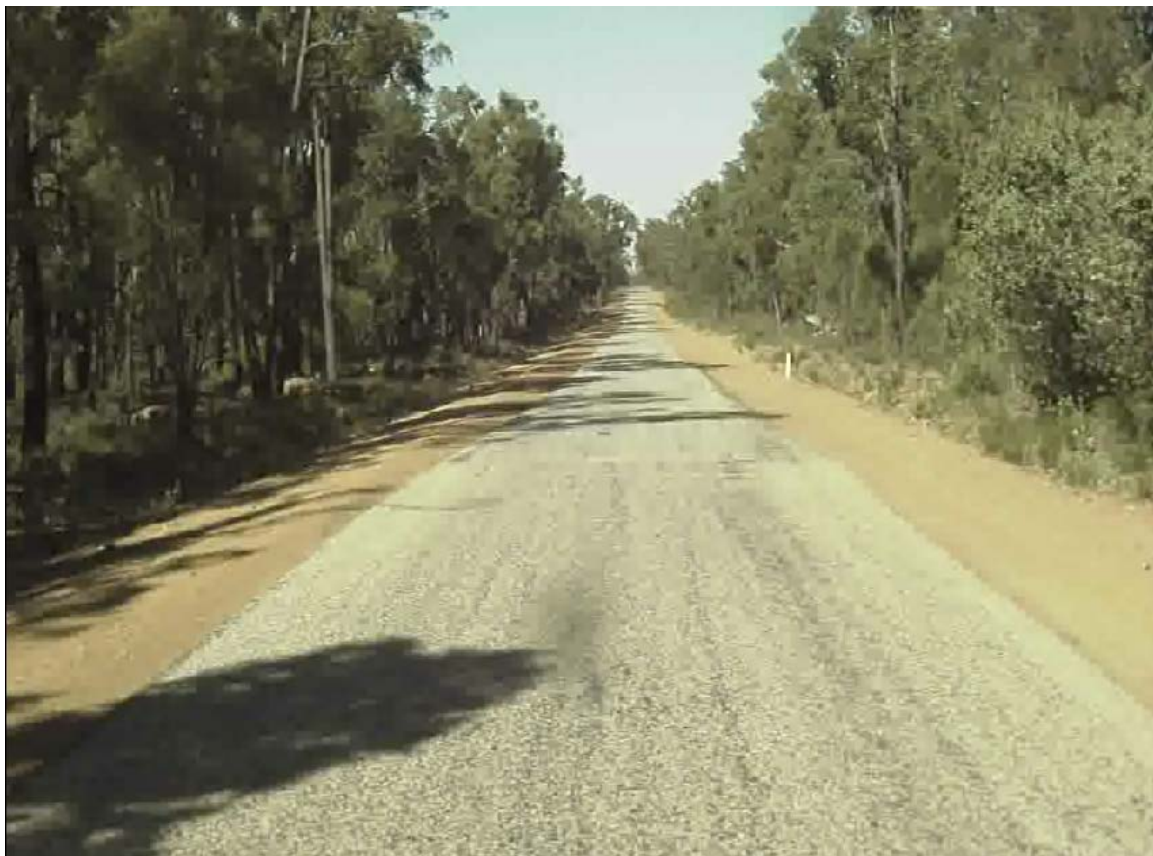
Plate 4 View north of road and road verge at 86.48 SLK
