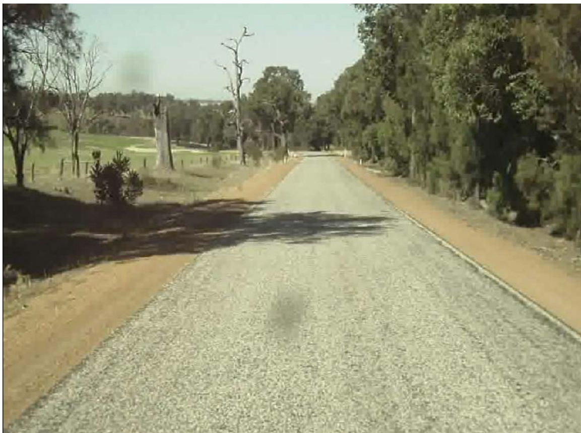
Plate 5 View north of road and road verge at 87.58 SLK
