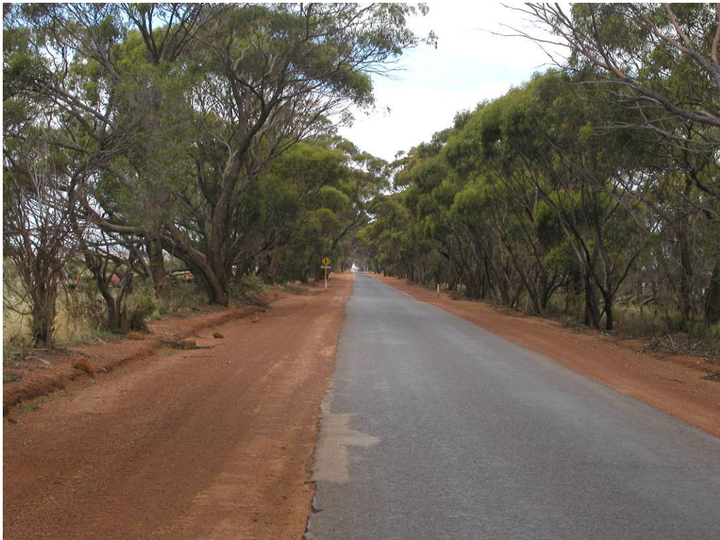
Figure 12: Existing road exiting Gorge Rock, to be widened (222.8 SLK facing east). Left side only to be cleared.
