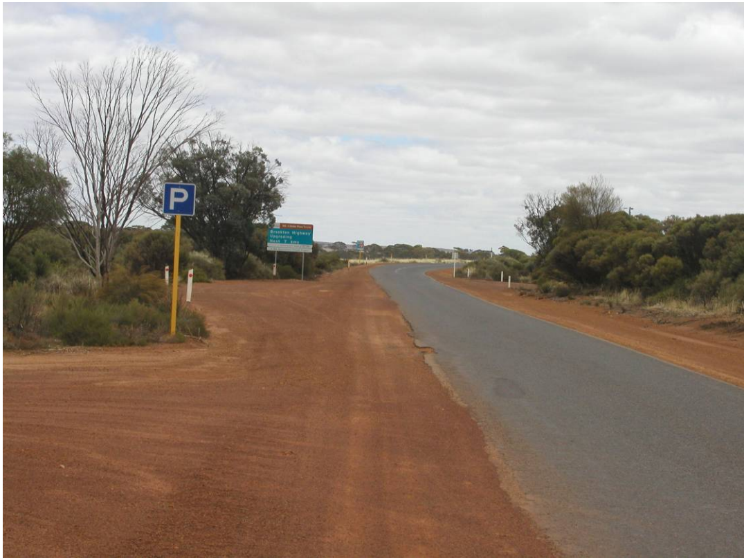
Figure 11: Existing Gorge rock alignment, to be closed (221.9 SLK facing west).
