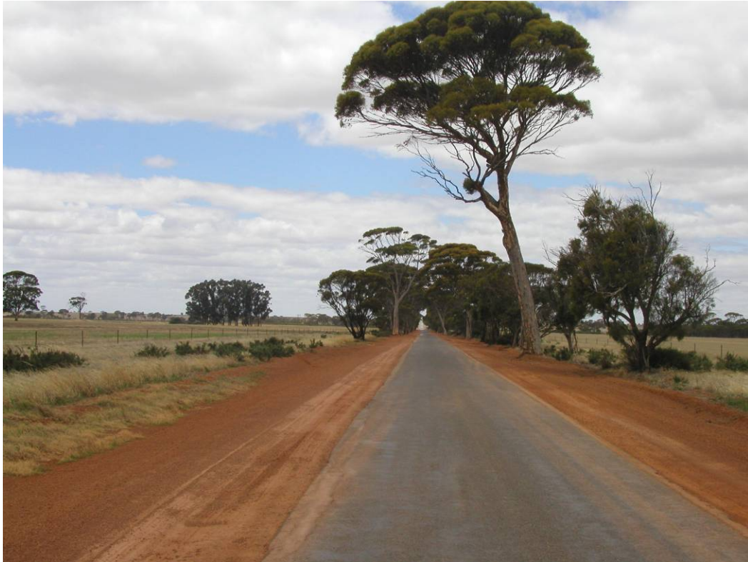
Figure 13: Existing road, Kondinin end, to be widened (224.8 SLK facing east). Left hand side only to be cleared.
