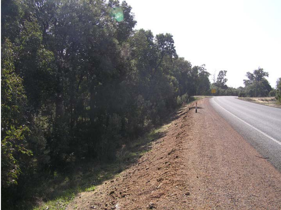
Northbound Carriageway, Bussell Highway, Facing North towards Harewoods Road
