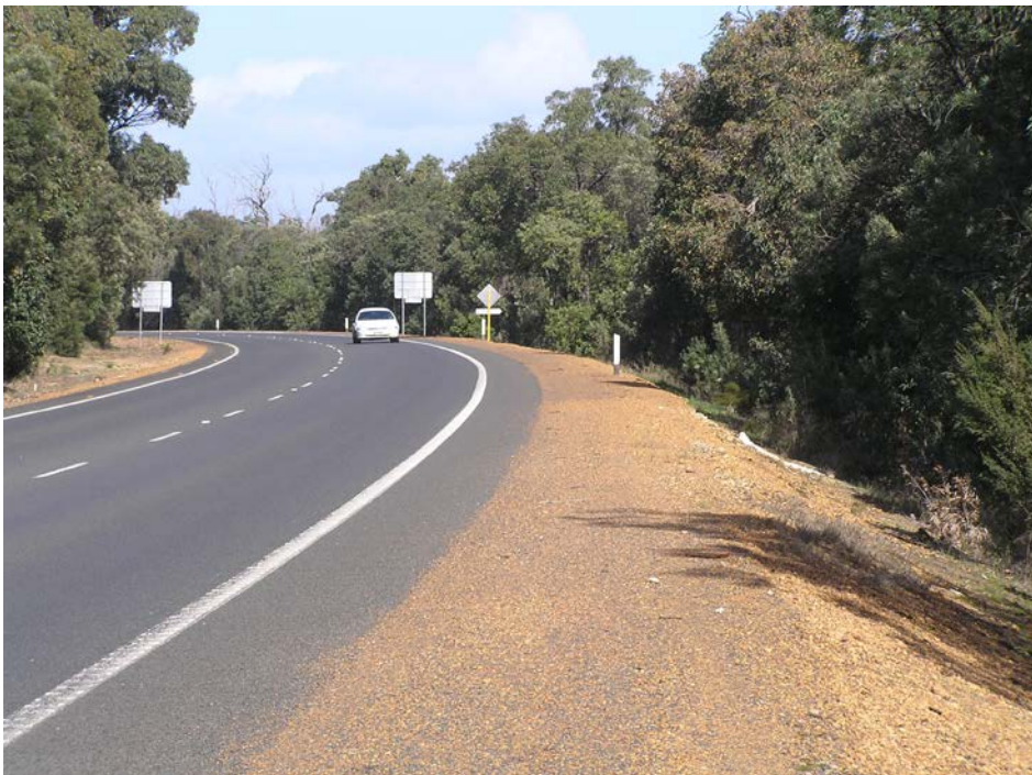
Location of Slip Lane, Northbound Carriageway, Facing South
