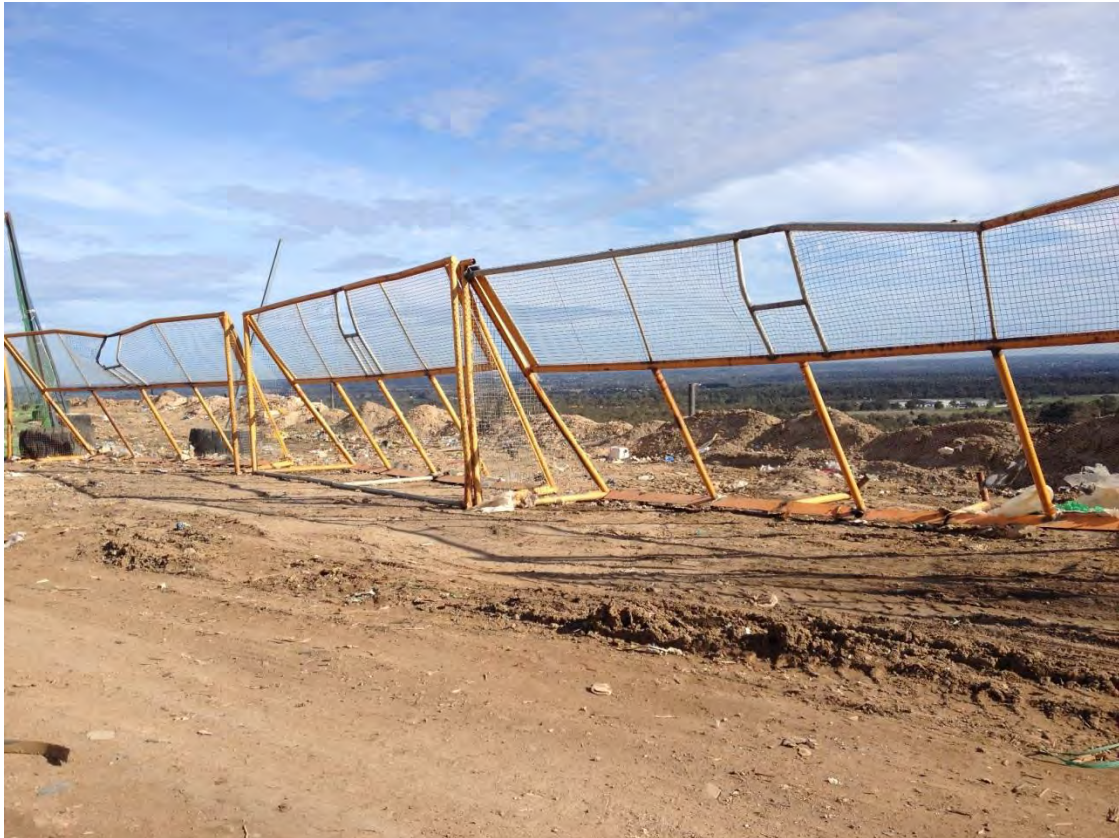
Figure 5: Litter-catching fence on top of daily cover.
