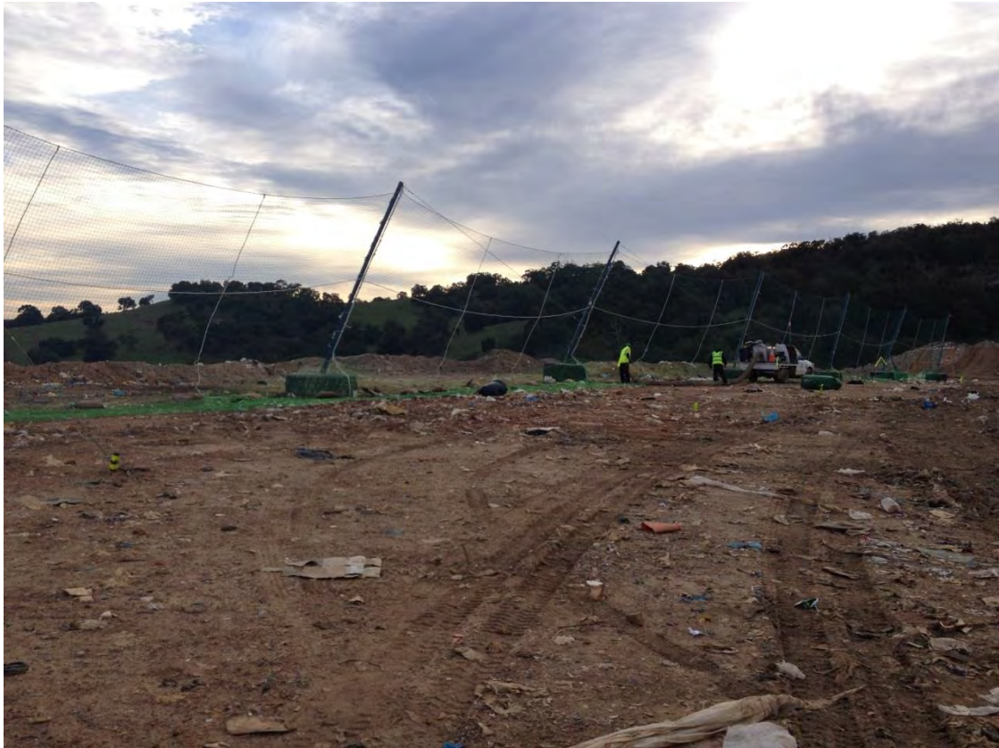
Figure 4: Temporary litter screens downwind from the active tipping face.
