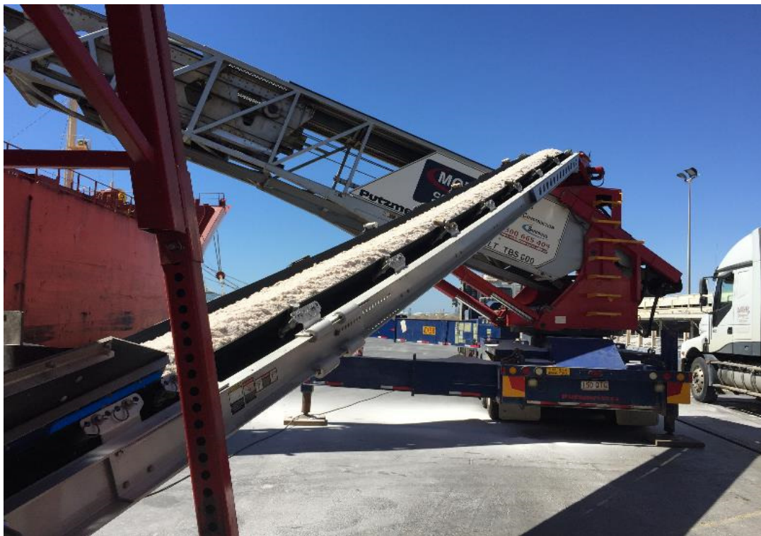
Conveyor belt changed from Chevron formation to flatter type to allow brush scrappers to be installed which eliminates carry back of material generating dust and spillage
