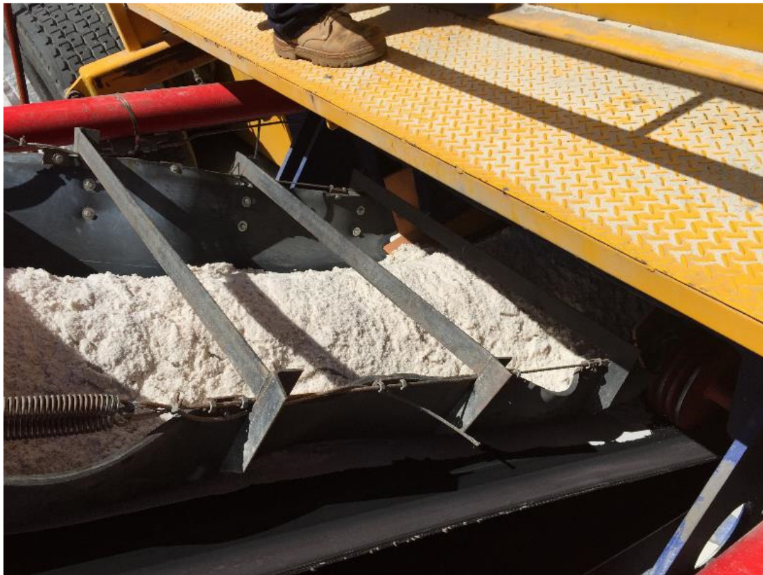
Hopper chute modified to place material in a heaped central piled, rather than a wide formation, in to reduce spillage off belt
