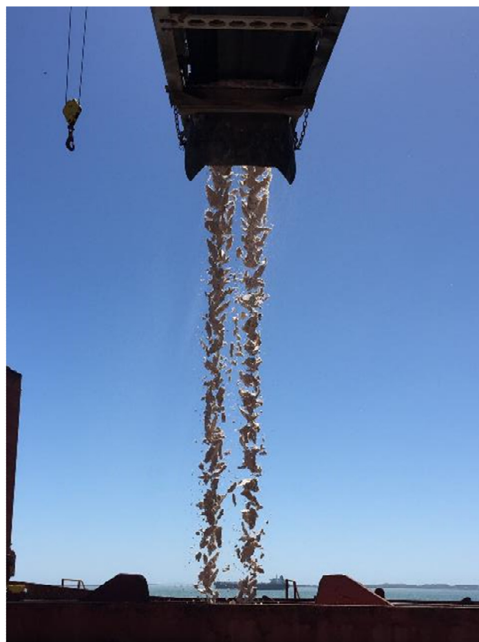
Shroud placed on the end of ship loader to reduce spillage and dust emissions
