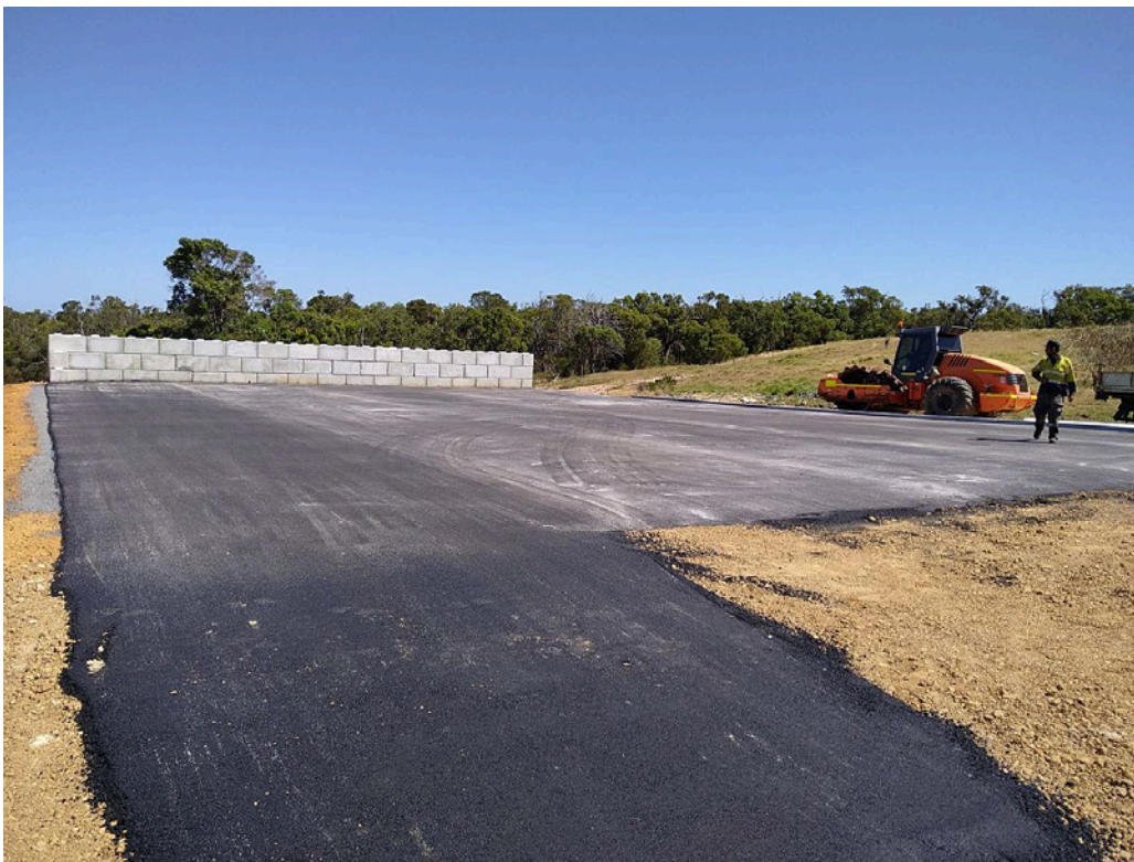
Figure 7: Fully Sealed hardstand
