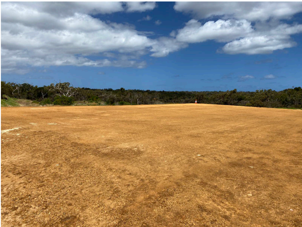
Figure 5: Prepared hardstand prior to sealing
