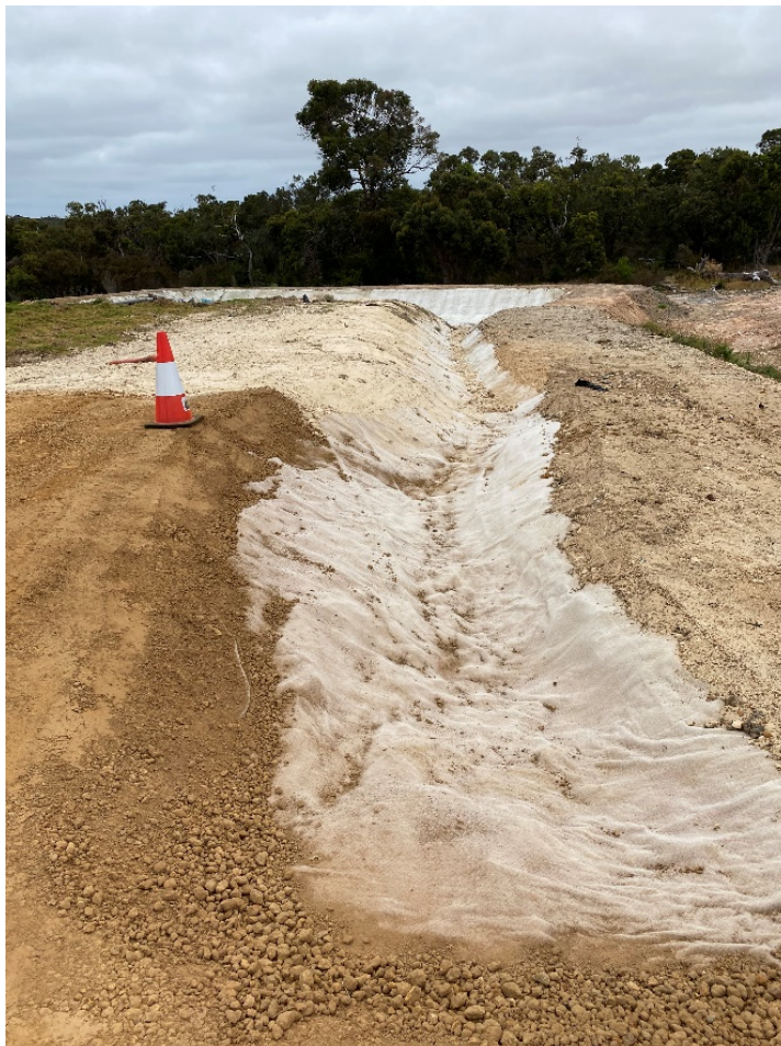
Figure 8: lined drainage channel
