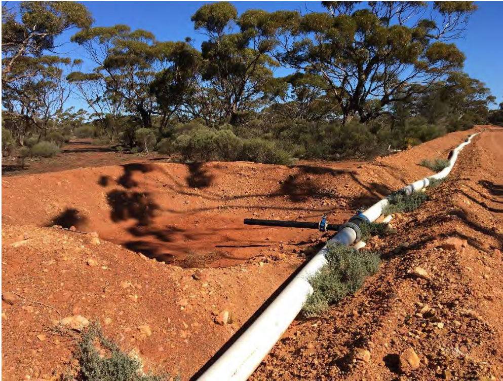
Figure 2: Pipeline maintained within a v-notch drain and catch sump / scour pit
