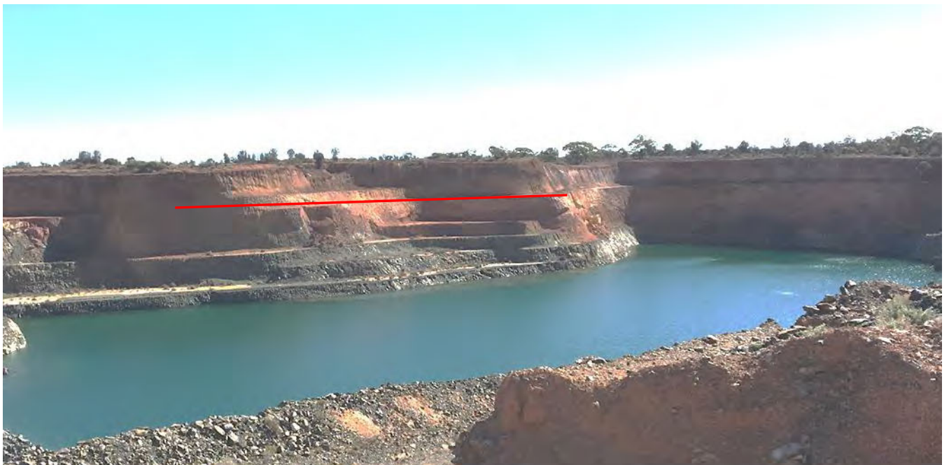
Figure 16: Lady Gladys Pit Lake on 20 June 2025. The 10m freeboard limit is indicated with the red line.
