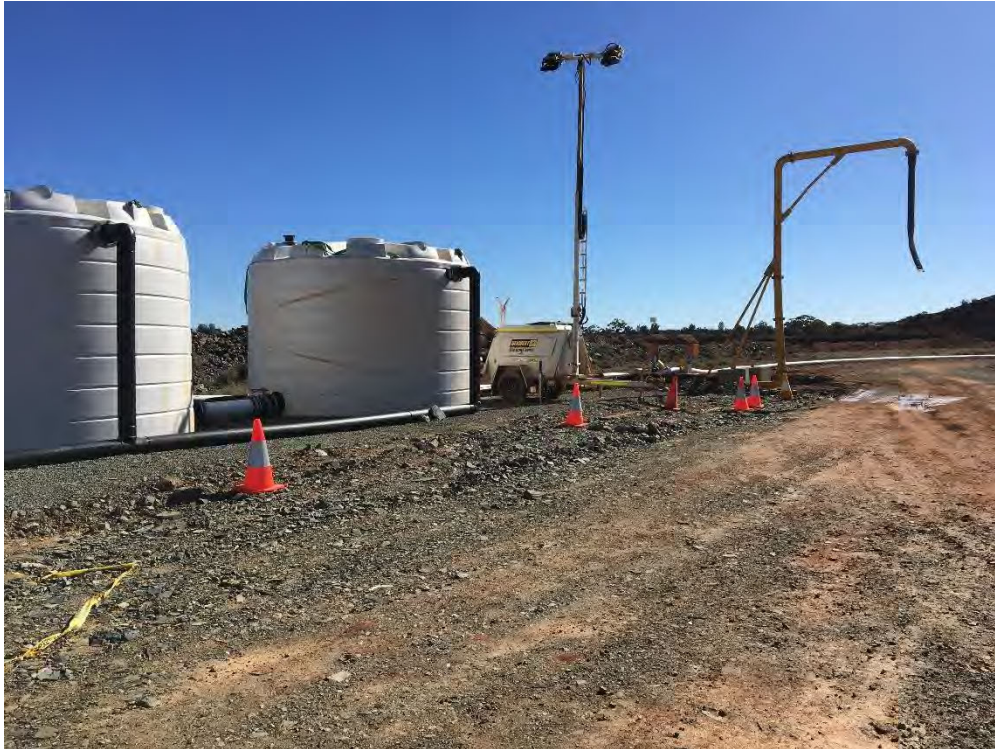
Figure 4: Infrastructure at the Lady Gladys Open Pit and Standpipe
