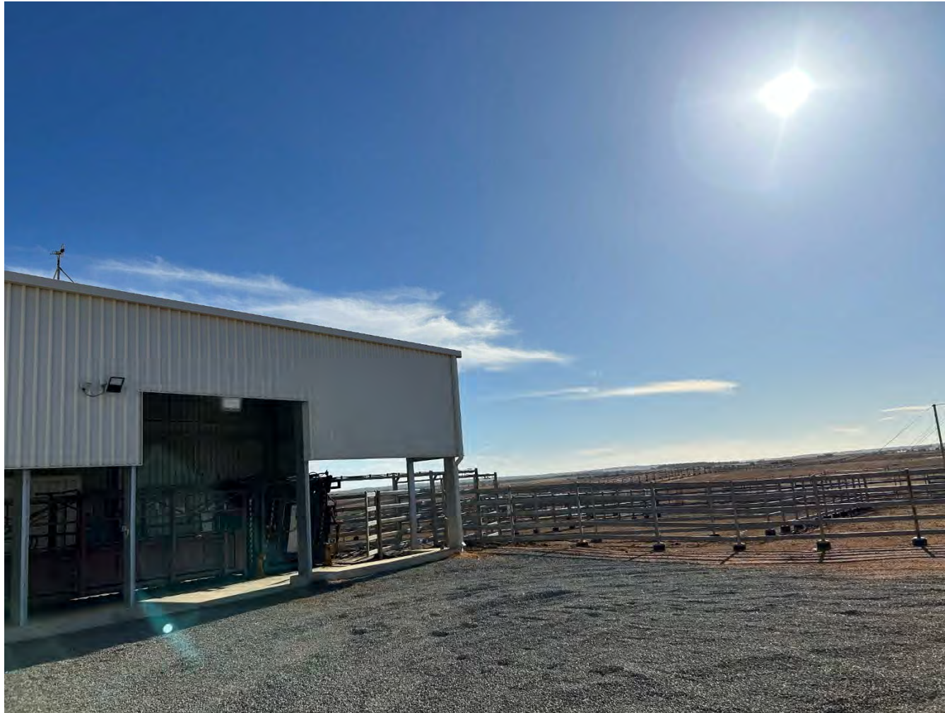
Photograph 1 – KDFP – Cattle handling facility
