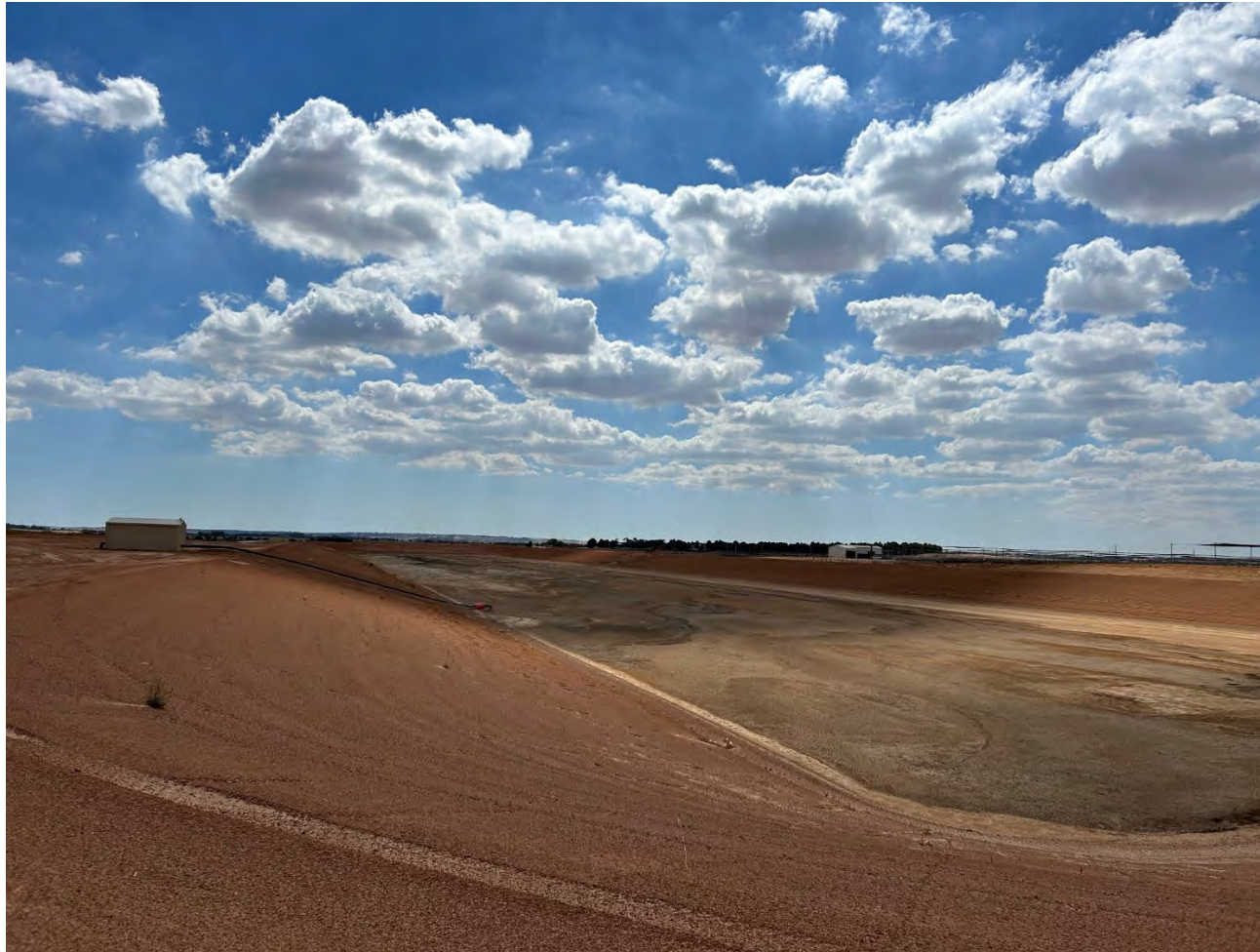
Photograph 5 – KDFE – Effluent Holding Pond 1
