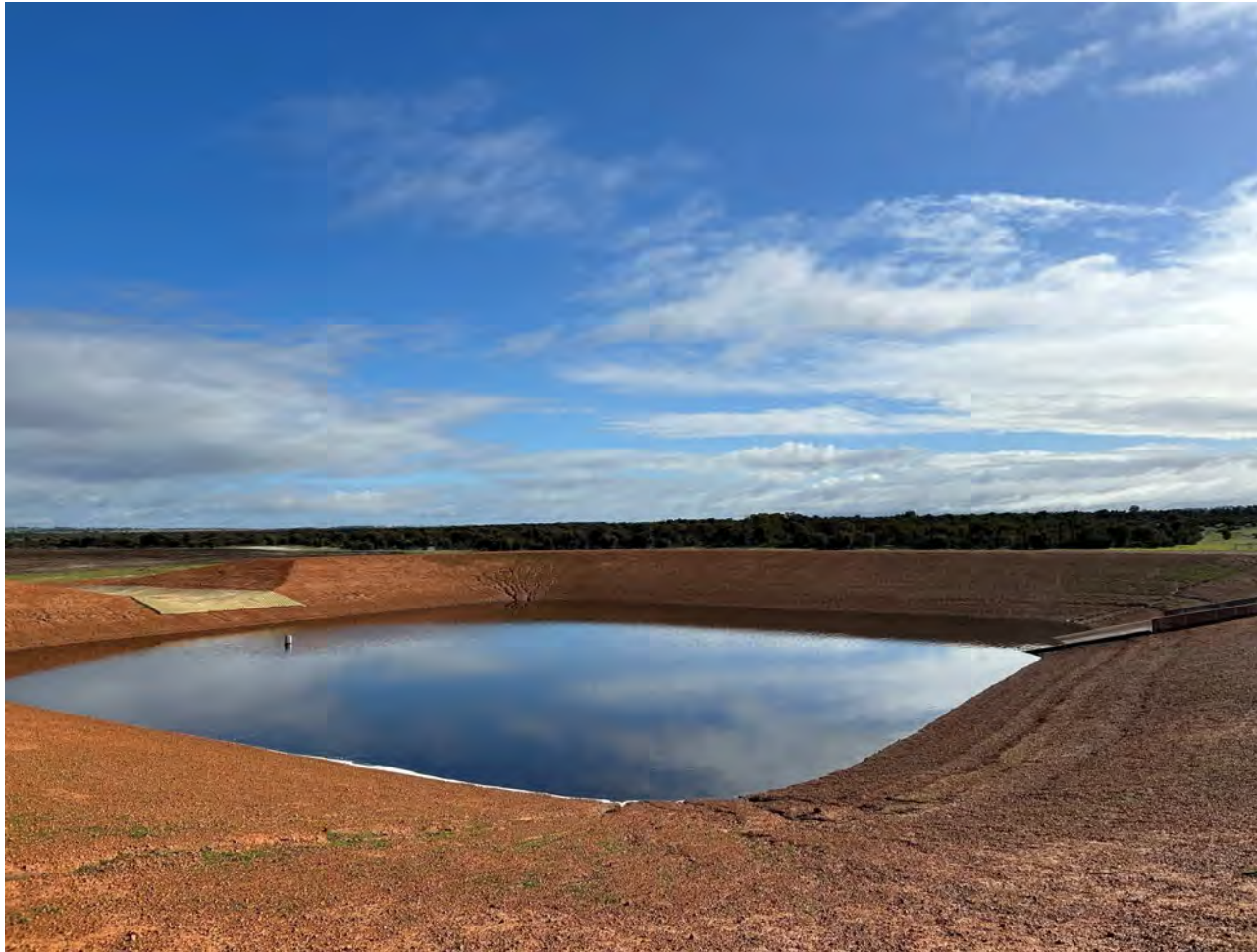
Photograph 8 – KDFE – Effluent Holding Pond 2
