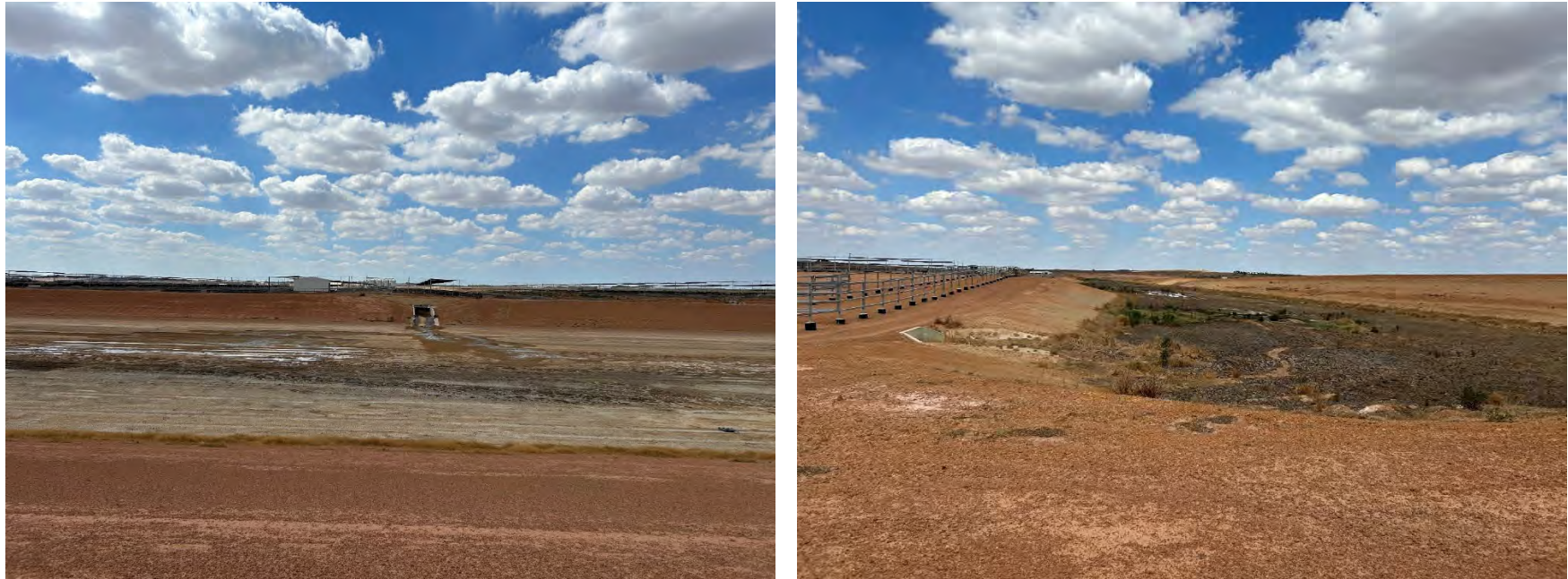
Photograph 4 – KDFP – Sedimentation basin 2 & 3 and control outlet weir
