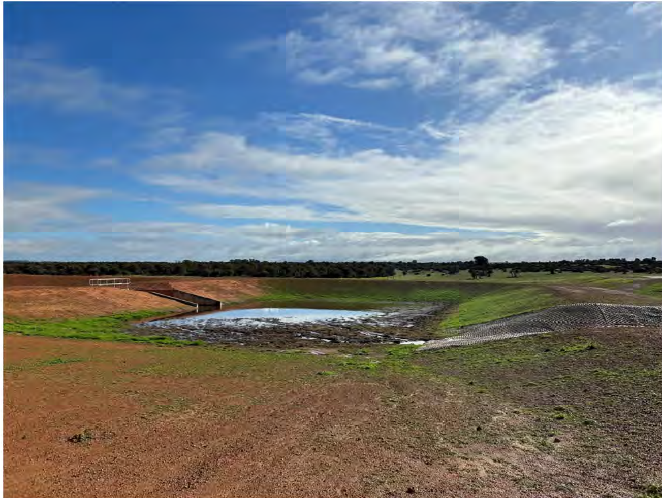
Photograph 7 – KDFP – Sedimentation basin 4 and control out weir
