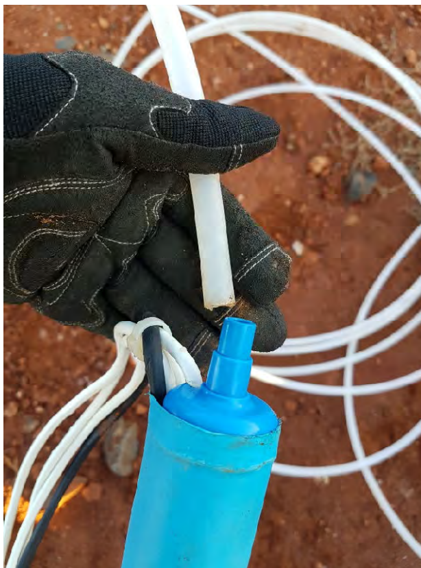
Photograph 3: Attach hose to pump.
