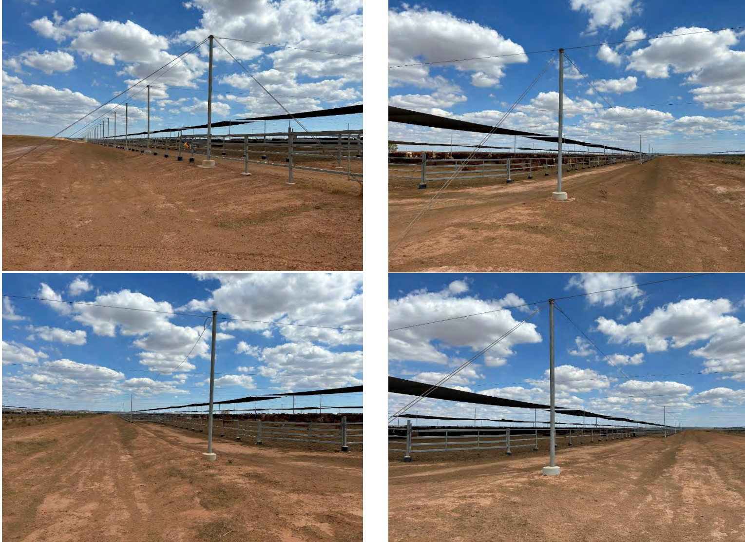
Photograph 3 – KDFE – Production pen effluent catch drains
