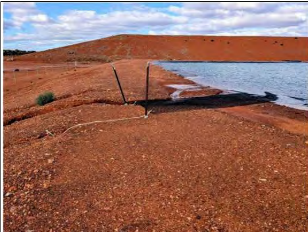
Figure 3: Turkey's Nest overflow point (22/06/2025)
