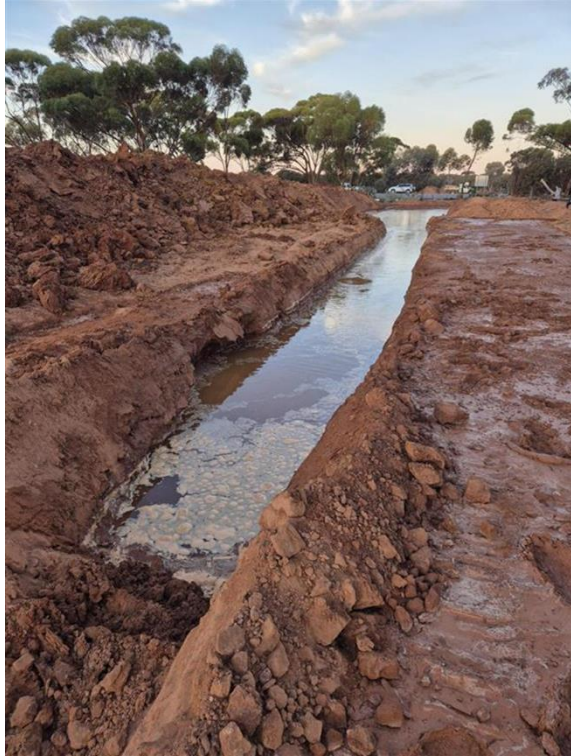
Photo-01 – Release water contained within the trench line
