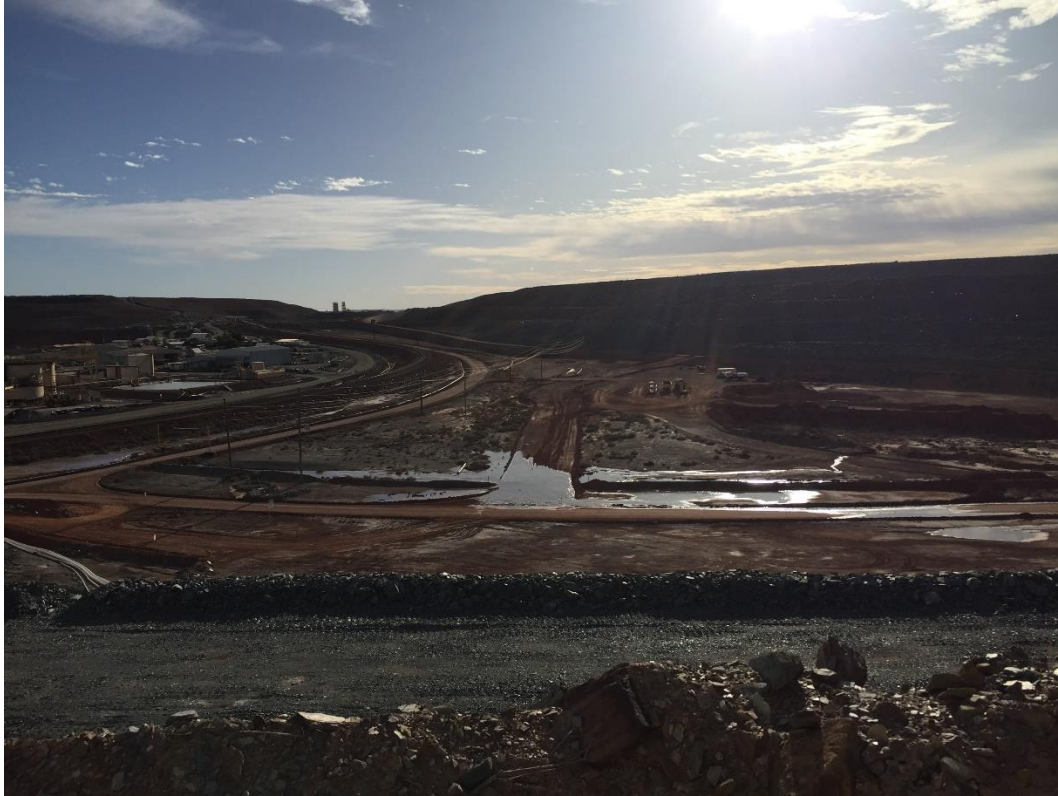
Plate 1. Tailings discharge outside of contained area.
