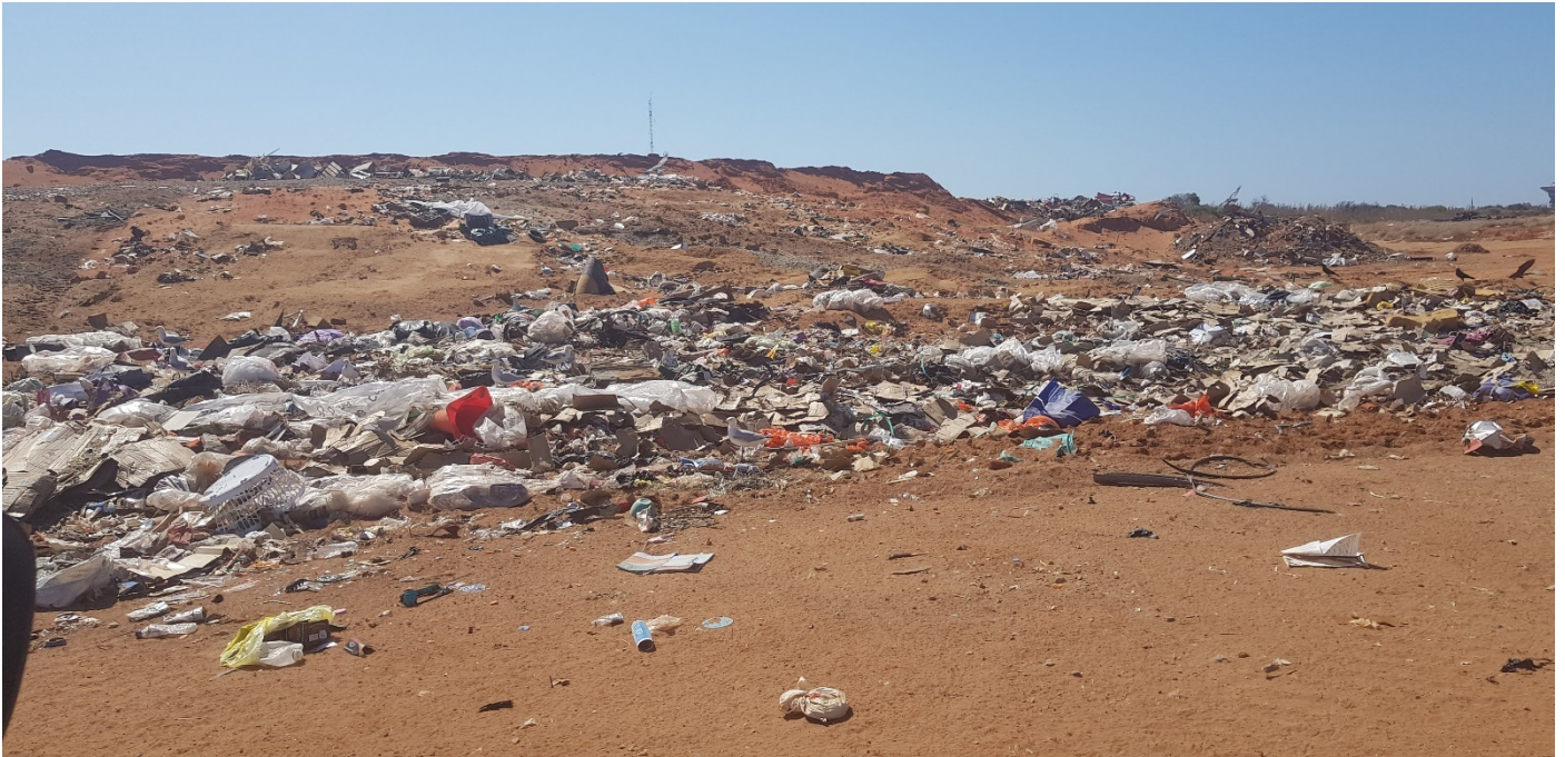
Figure 8. This is the old publicly accessible putrescible area which could use some improvement. This area is more prone to windblown waste blowing sideways. It is recommended to phase this out now that public entry is predominantly limited to the skip bins.
