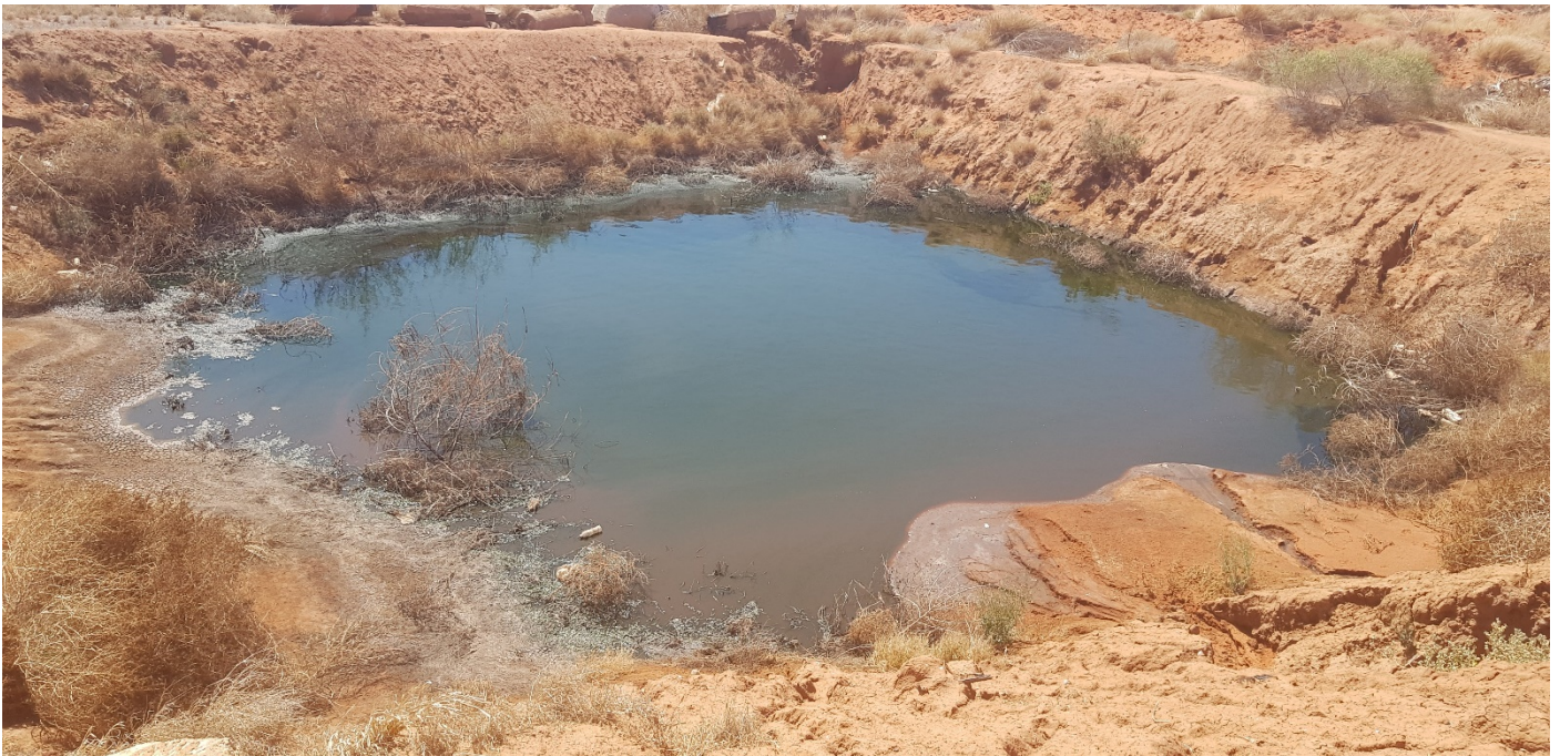
Figure 4. Liquid waste is increasing and a new location and design is recommended. Currently there are 2 primary pits and 2 secondary pits but the secondary pits should be larger and shallower to promote more evaporation, and all should be further from the tip entrance to reduce odour. Ideally the tip entrance and buildings would be on the southern side of the premises (upwind) but they are currently directly downwind of the liquid waste ponds.
