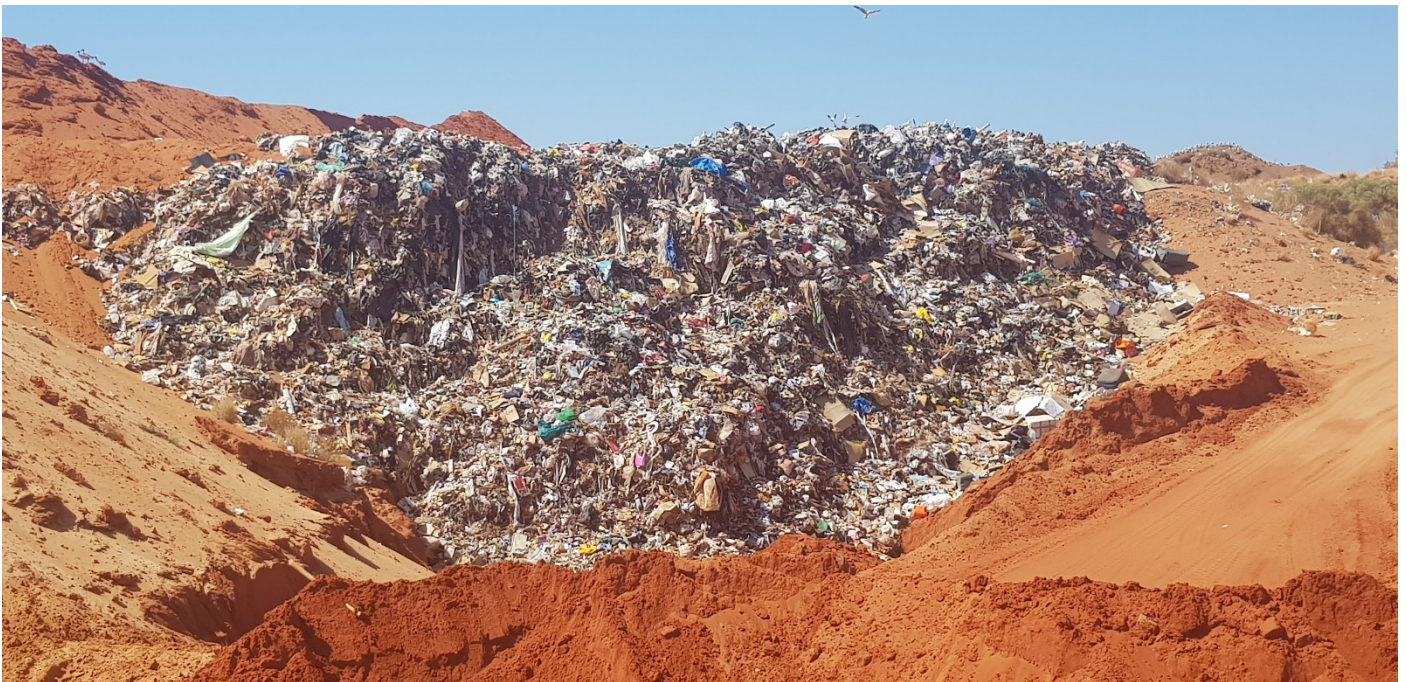
Figure 7. Putrescible area was being covered on the top during the inspection. There was very little wind blown waste on top and no obvious odour. The prevailing wind blows into the face.
