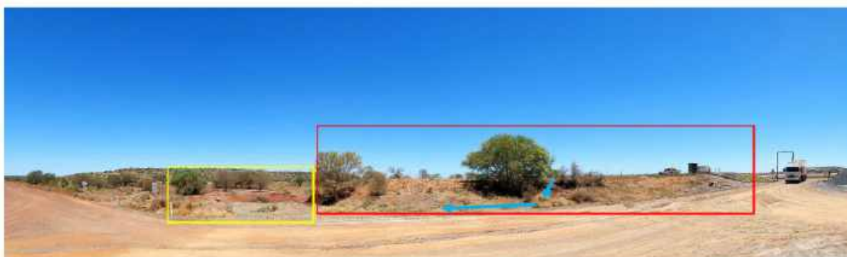
Figure 1: shows the Main Turkeys Nest Dam within the red square, and location of overflow with approximate extent of spillage highlighted by blue arrows. The yellow square highlights the road drainage sump adjacent to the Main Turkeys Nest Dam.
