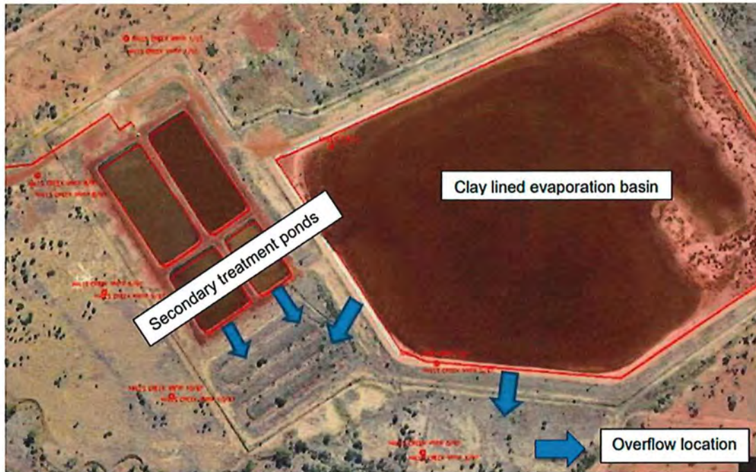
Figure 1: Halls Creek Wastewater Treatment Plant Overflow Locations
