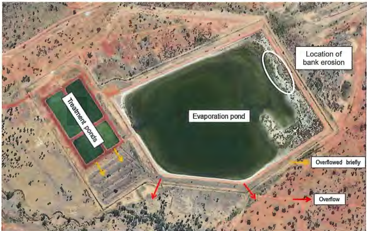
Figure 1: Halls Creek Wastewater Treatment Plant Discharge Points and Bank Erosion
