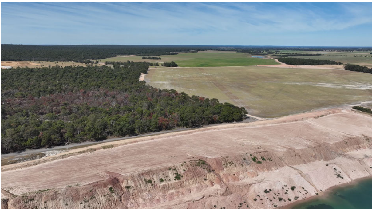
Plate 2 – Stockpiled material for future capping of 90ft Pit.
