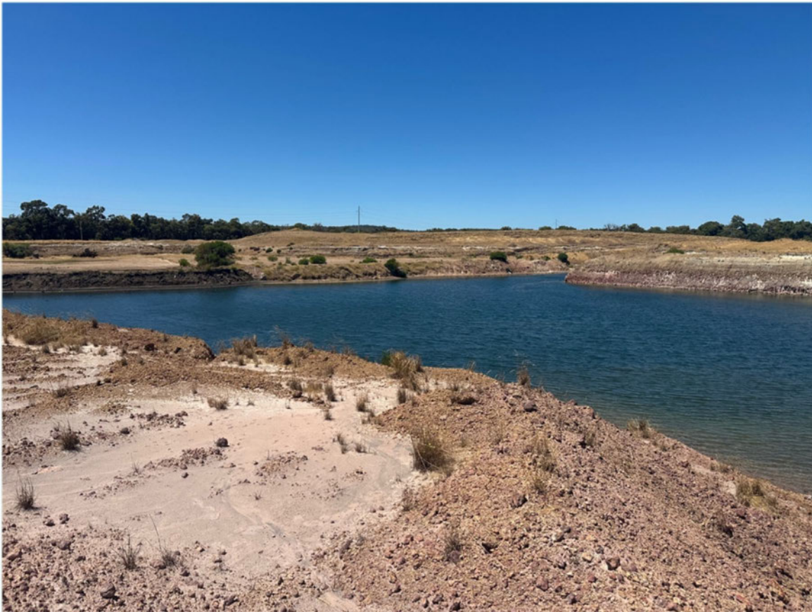
Plate 1 - 90ft Waste Disposal Pit, February 2025.
