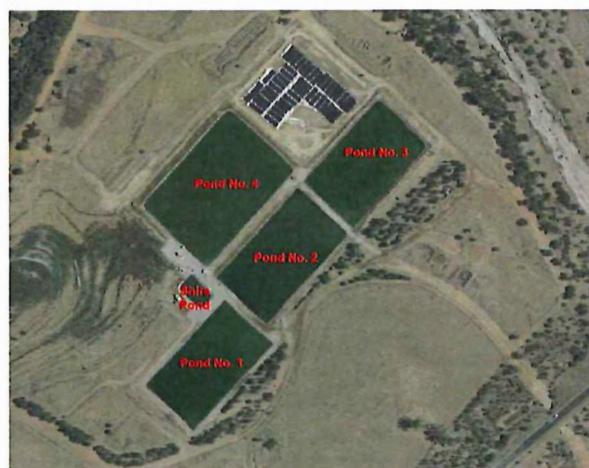
Figure 1. Aerial of Northam WWTP
