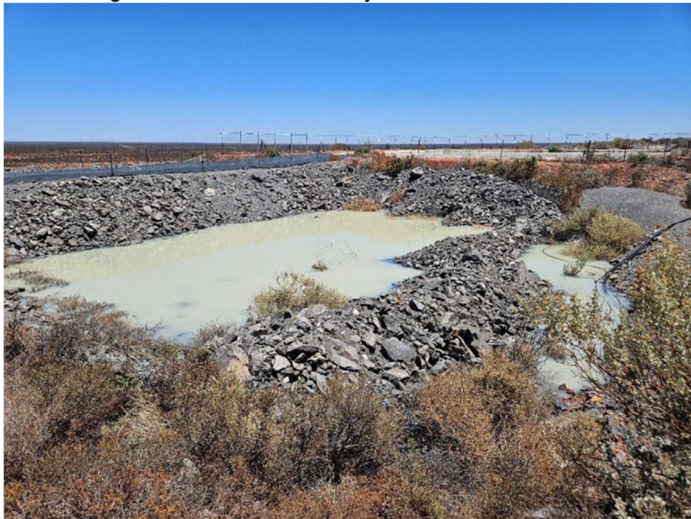
Figure 4 - New Holland Turkeys nest overflow old sediment sump.
