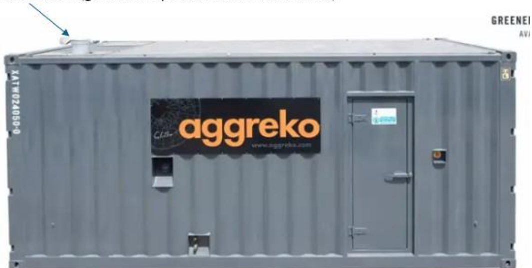
Figure 4 Exhaust point on each containerised generator
