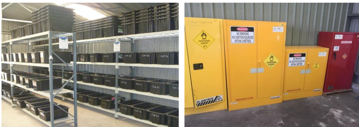
Figure 1: Example segregated storage racking and receptacles (left) and dangerous goods cupboards (right)
