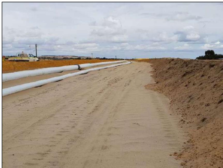
▲ *Figure 11: Example of secondary containment to be constructed for all pipelines.*
