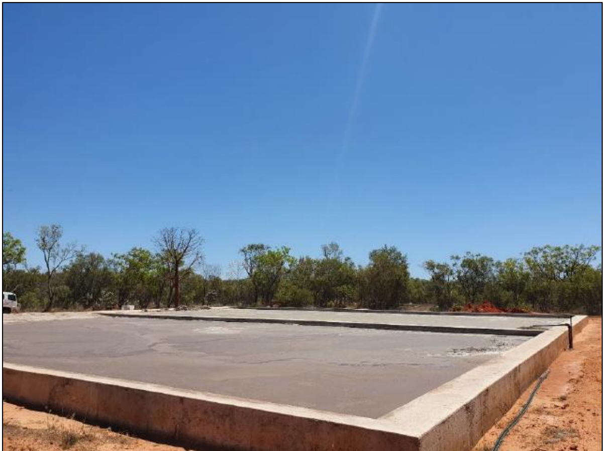
Figure 2: Constructed concrete brine evaporation pads
