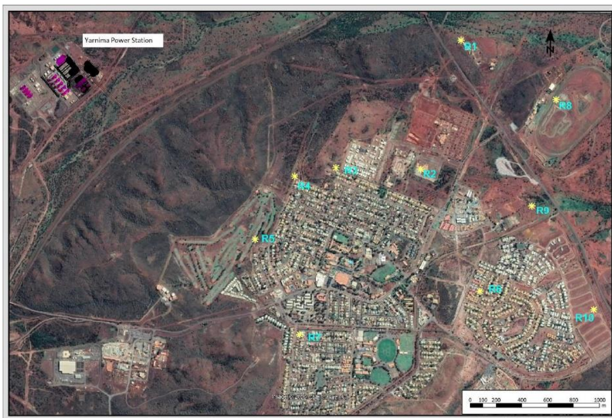
Figure 1: Location of Yarnima Power Station and noise sensitive receptors.
