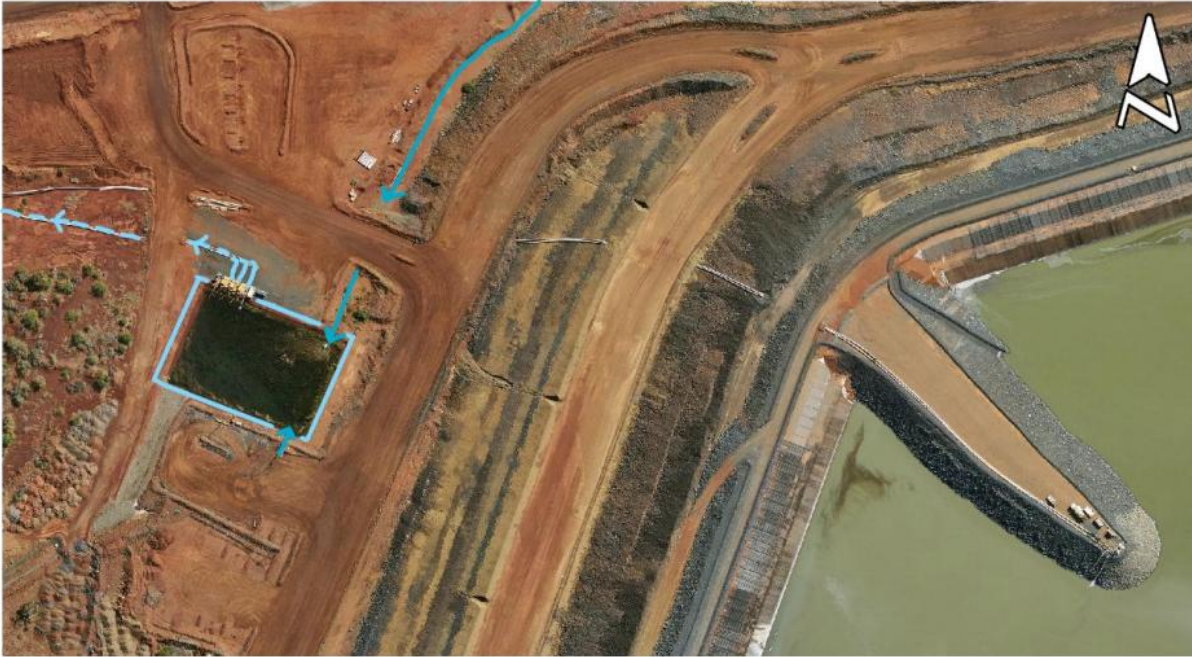
Figure 3: Seepage collection pond
