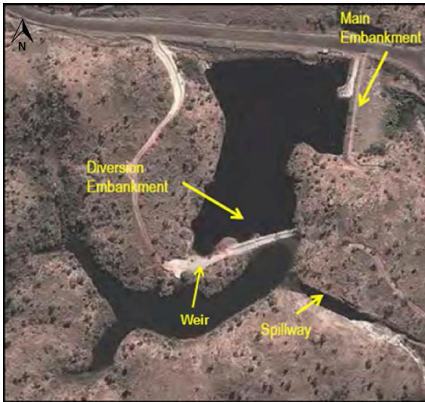
Figure 1: WSF1 and Spillway
