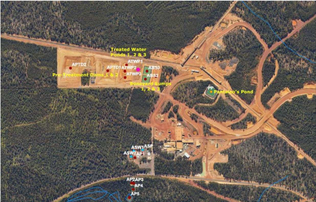
Figure 4: Arundel mining area - sumps, pre-treatment dams and treated water ponds
