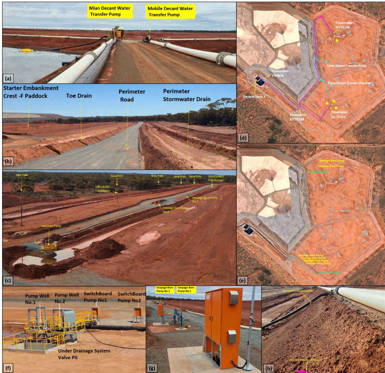
Figure 2: Photographs of FIM II TSF Cells E and F – (a) return water pipelines along decant accessway, (b) water management infrastructure, (c) water management infrastructure, (d) decant pump and return water pipeline layout, (e) underdrainage system, toe drainage and seepage recovery bore layout, (f) underdrainage sump, (g) pumps for seepage recovery bores, (h) freeboard marker on upstream embankment
