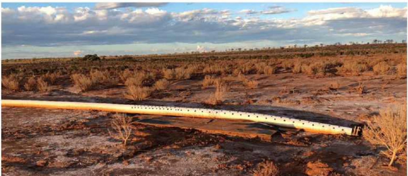
Plate 2: Example of Discharge Pipeline Baffling
