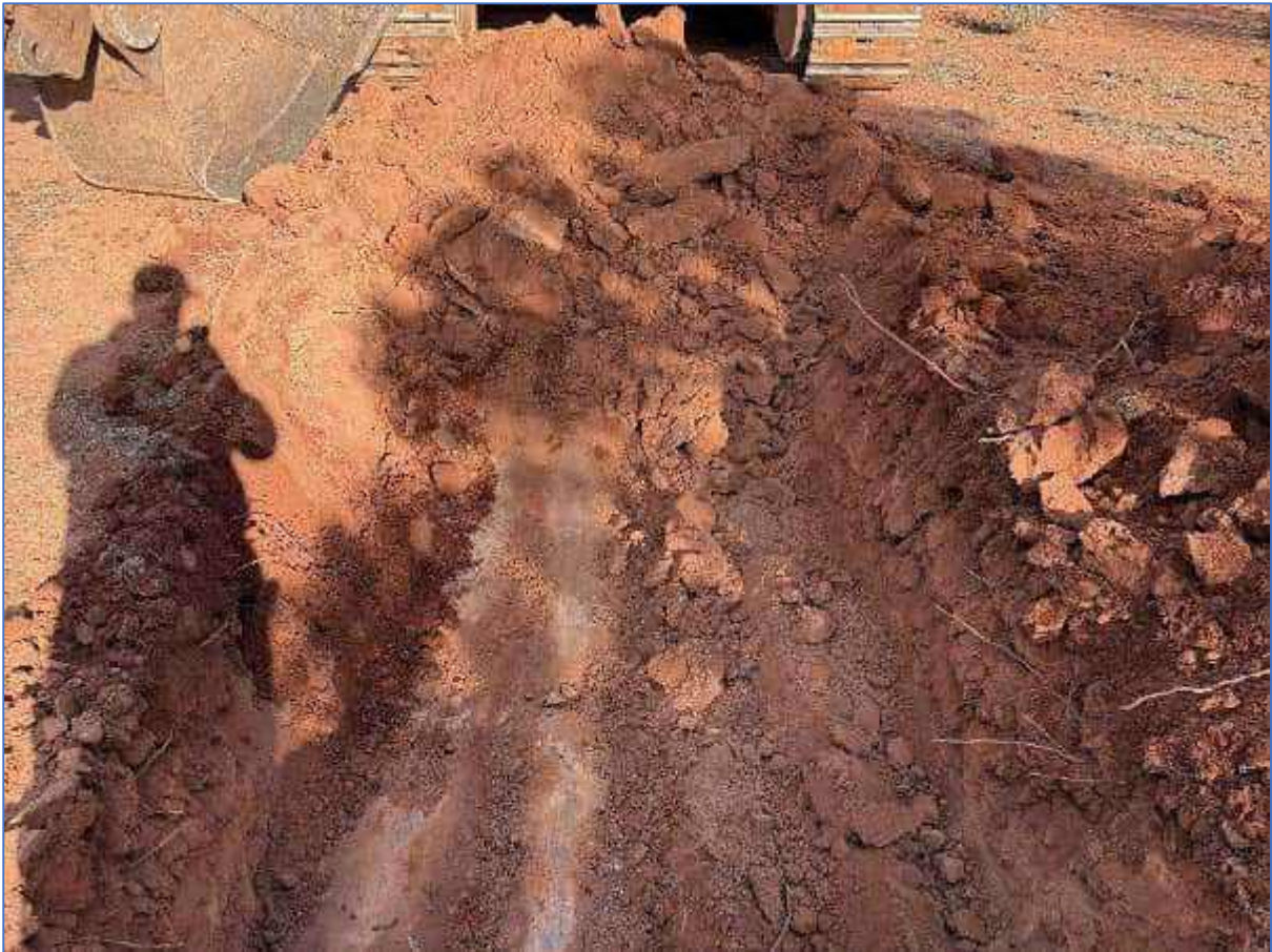
Plate 70: TSF-TP15 – Test Pit location
