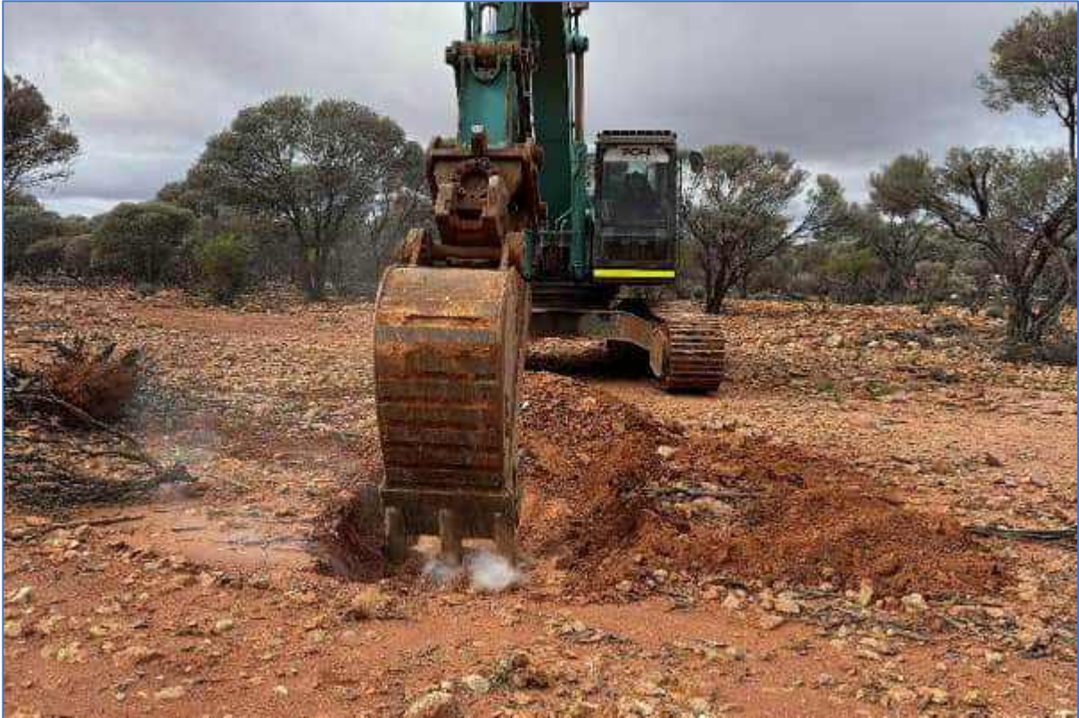
Plate 7: TSF-TP-02 – Test Pit location
