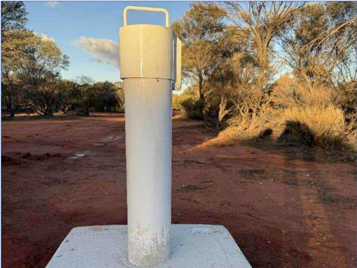
Plate 89: TSF-TP19 – Adjacent standpipe piezometer (TSF-BH03)
