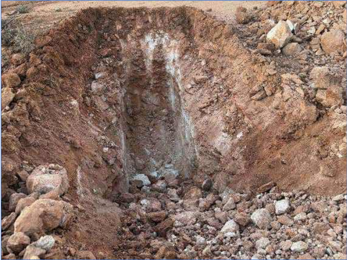
Plate 99: TSF-TP22 – Excavation to refusal
