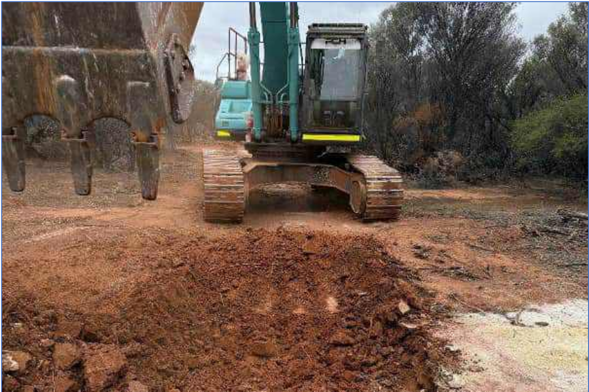
Plate 31: TSF-TP07 – Test Pit location
