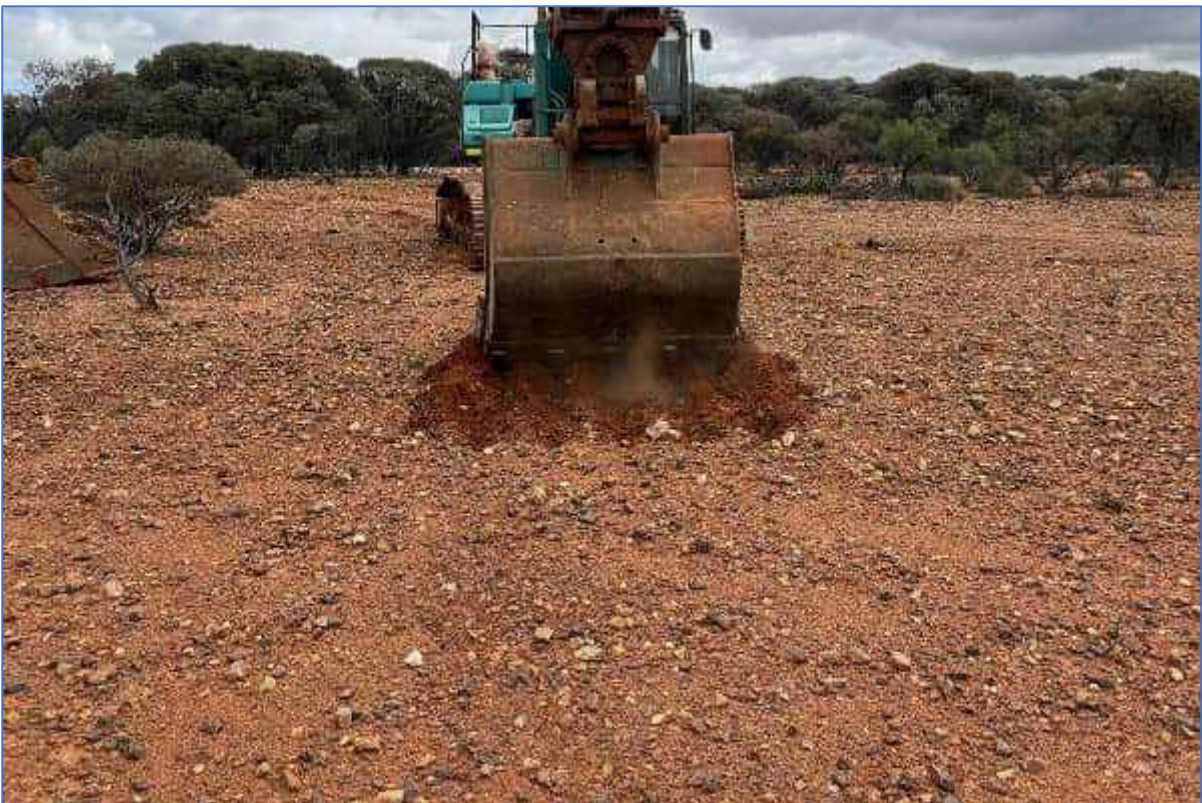
Plate 28: TSF-TP06 – Test Pit location
