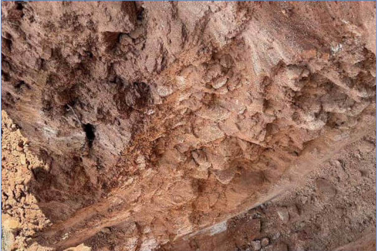
Plate 53: TSF-TP11 – Test Pit wall
