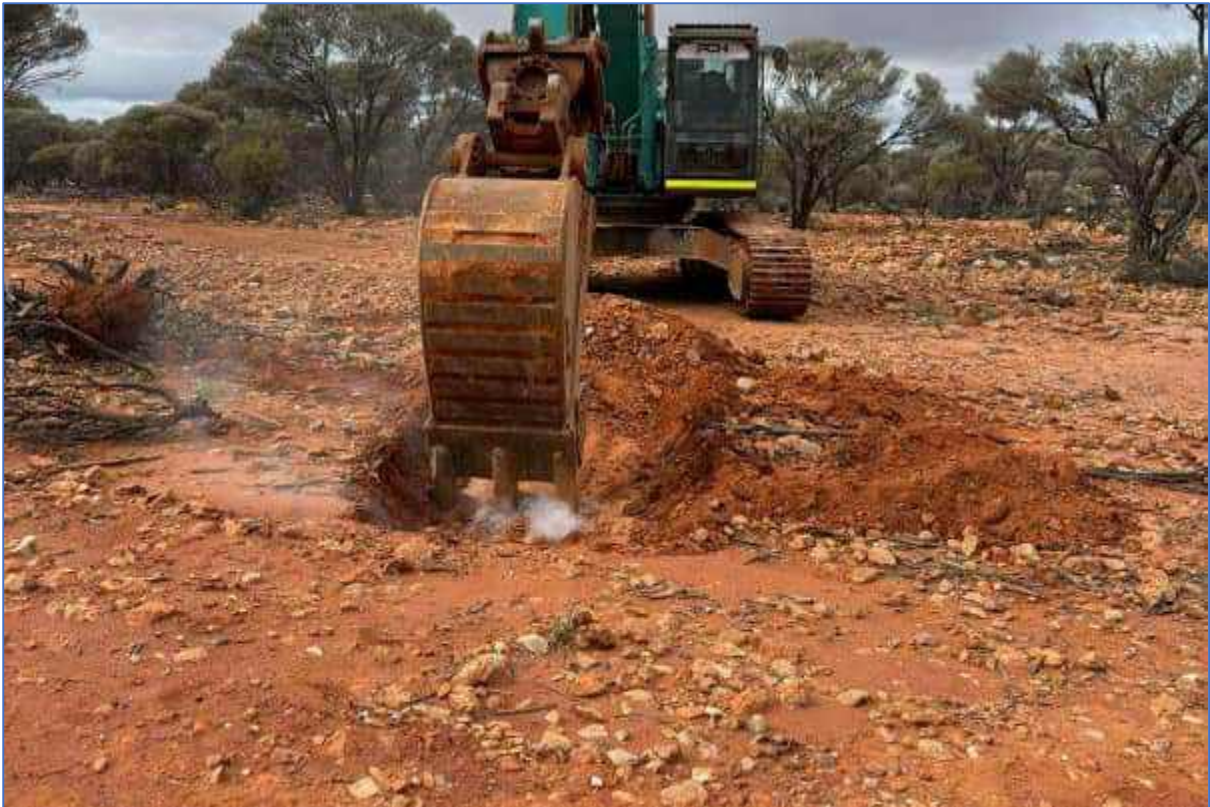
Plate 13: TSF-TP03 - Test Pit location
