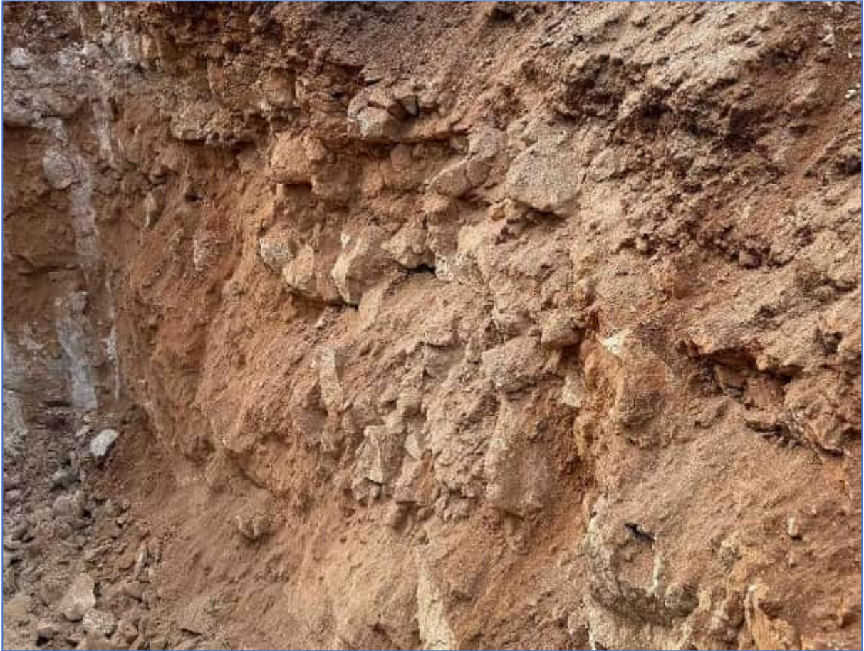
Plate 3: TSF-TP-01 – Excavation Wall
