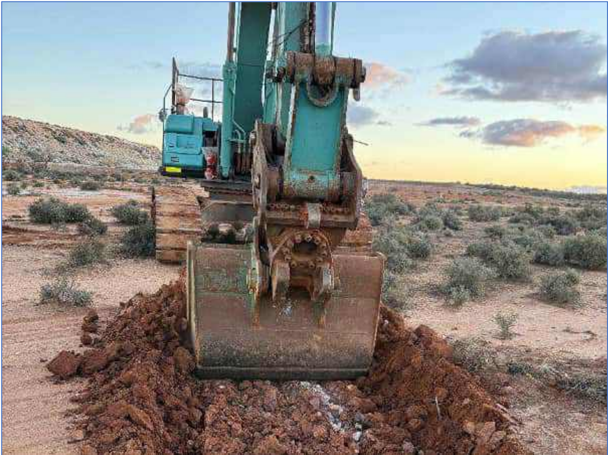
Plate 98: TSF-TP22 – Test Pit Location
