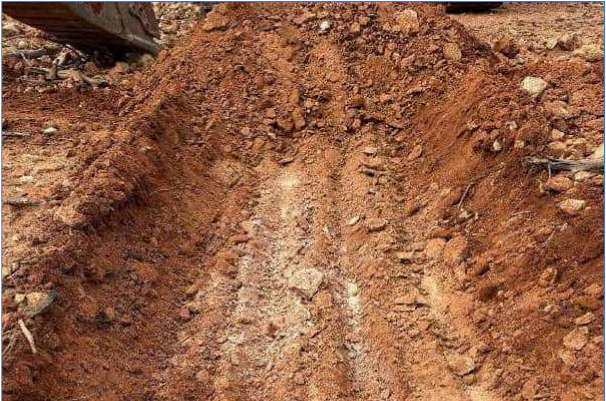
Plate 14: TSF-TP03 - Excavation to refusal
