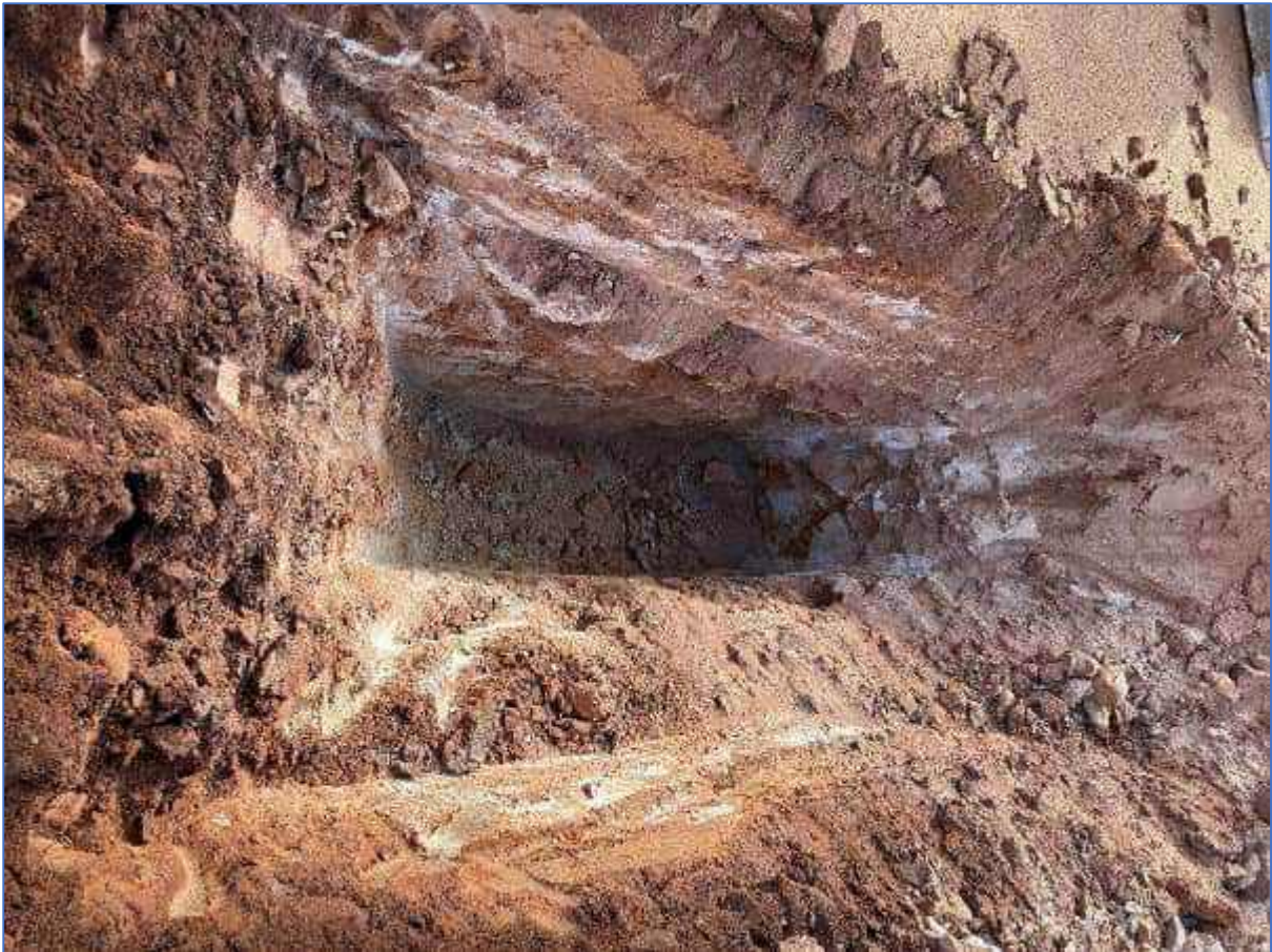
Plate 42: TSF-TP09 – Excavation to refusal
