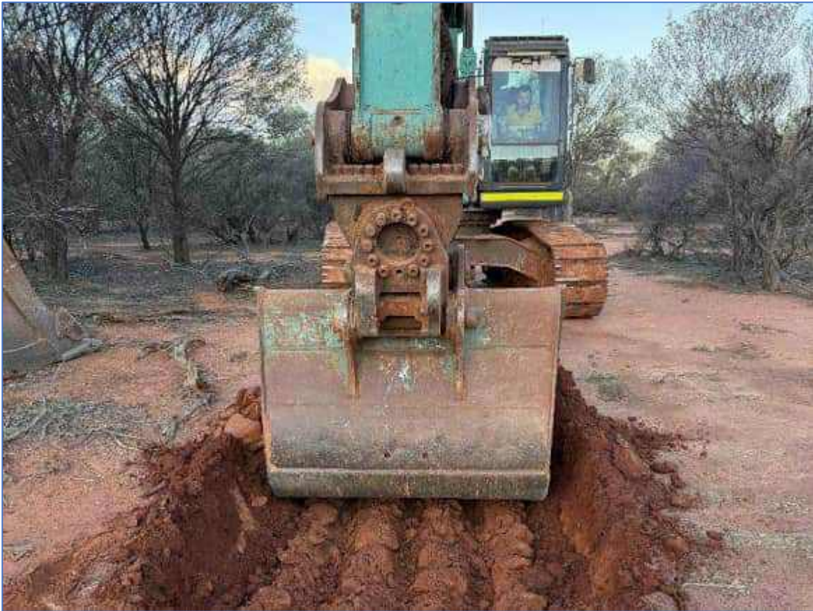
Plate 91: TSF-TP20 – Test Pit Location
