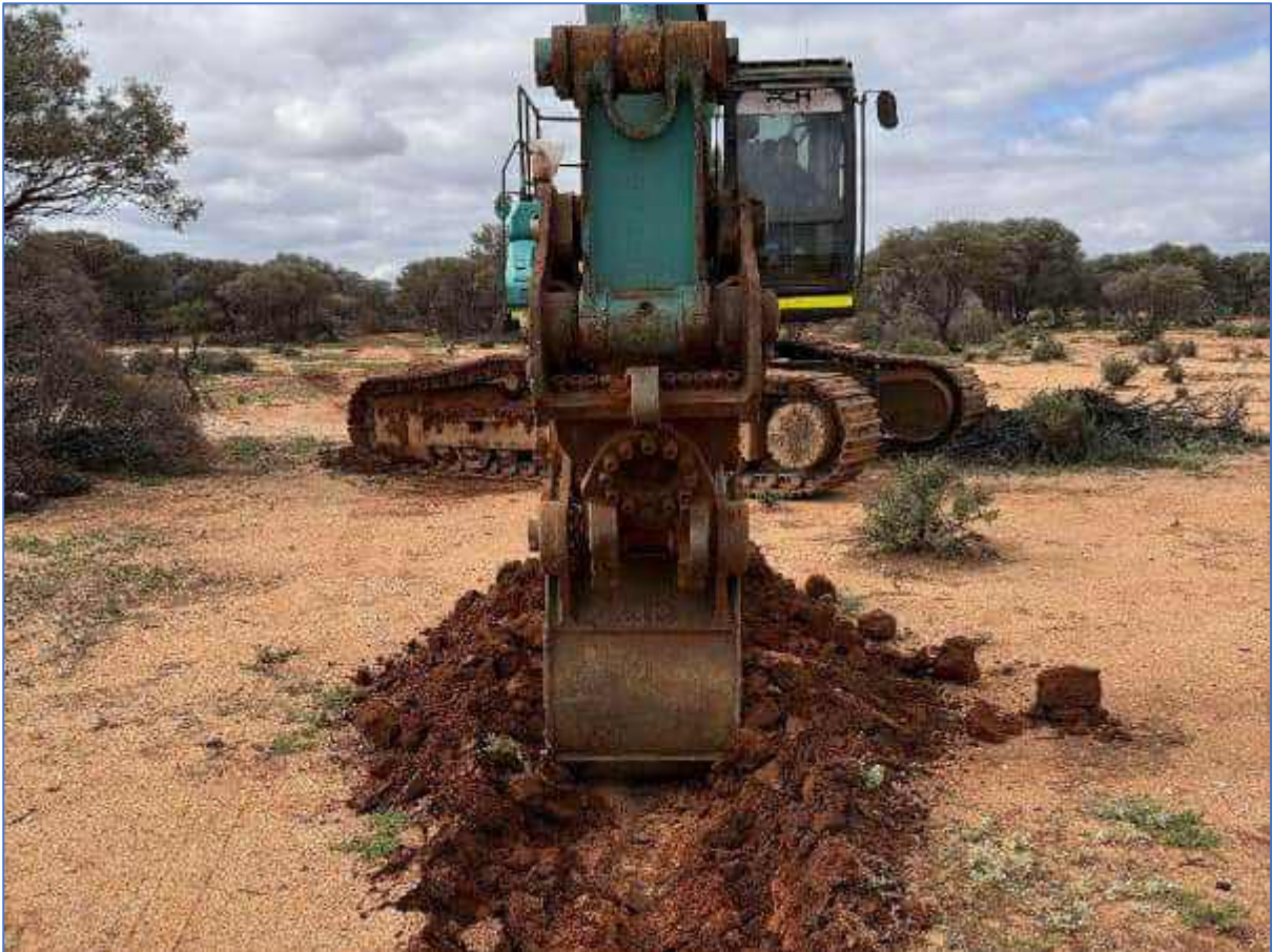
Plate 45: TSF-TP10 – Test Pit Location
