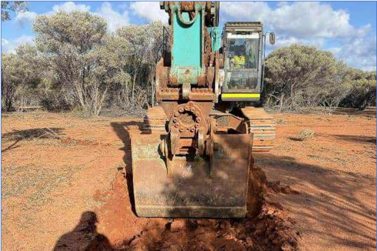
Plate 69: TSF-TP15 – Test Pit location
