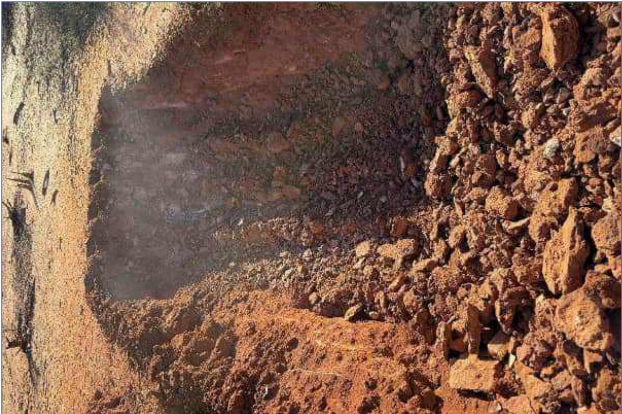
Plate 74: TSF-TP16 – Excavation to refusal
