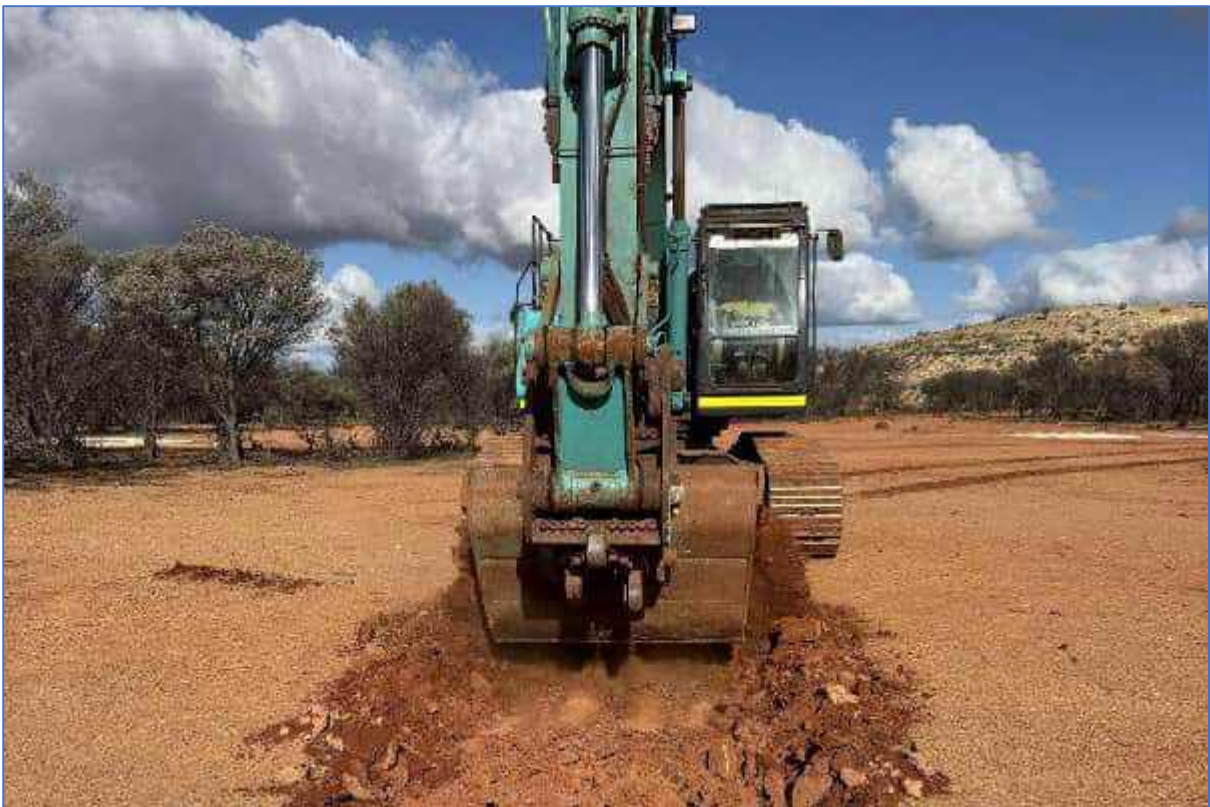
Plate 56: TSF-TP12 – Test Pit location
