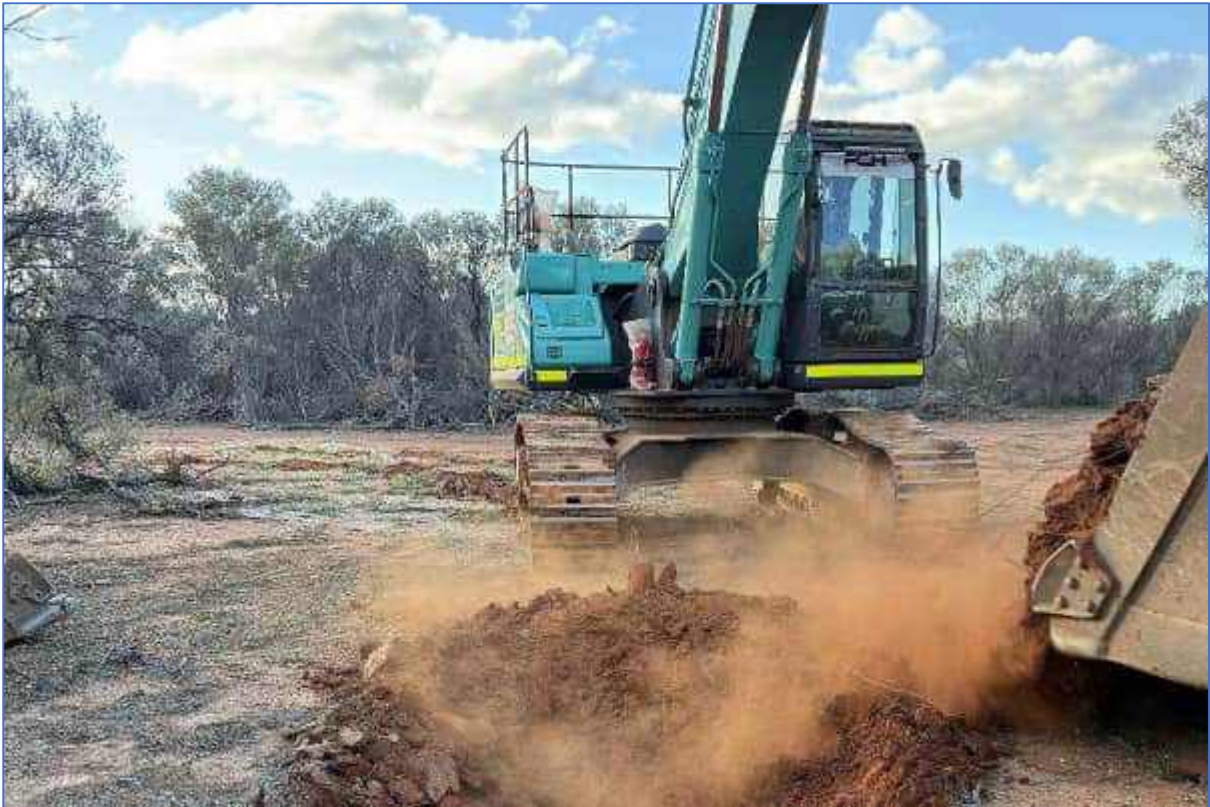
Plate 81: TSF-TP18 – Test Pit location
