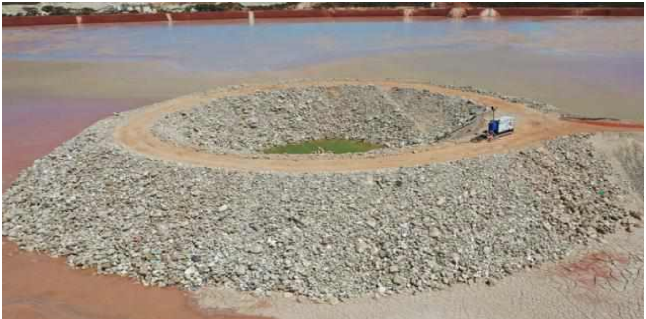
Figure 3-2: Typical rock ring decant arrangement
