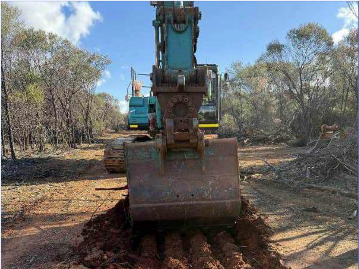
Plate 64: TSF-TP14 – Test Pit location
