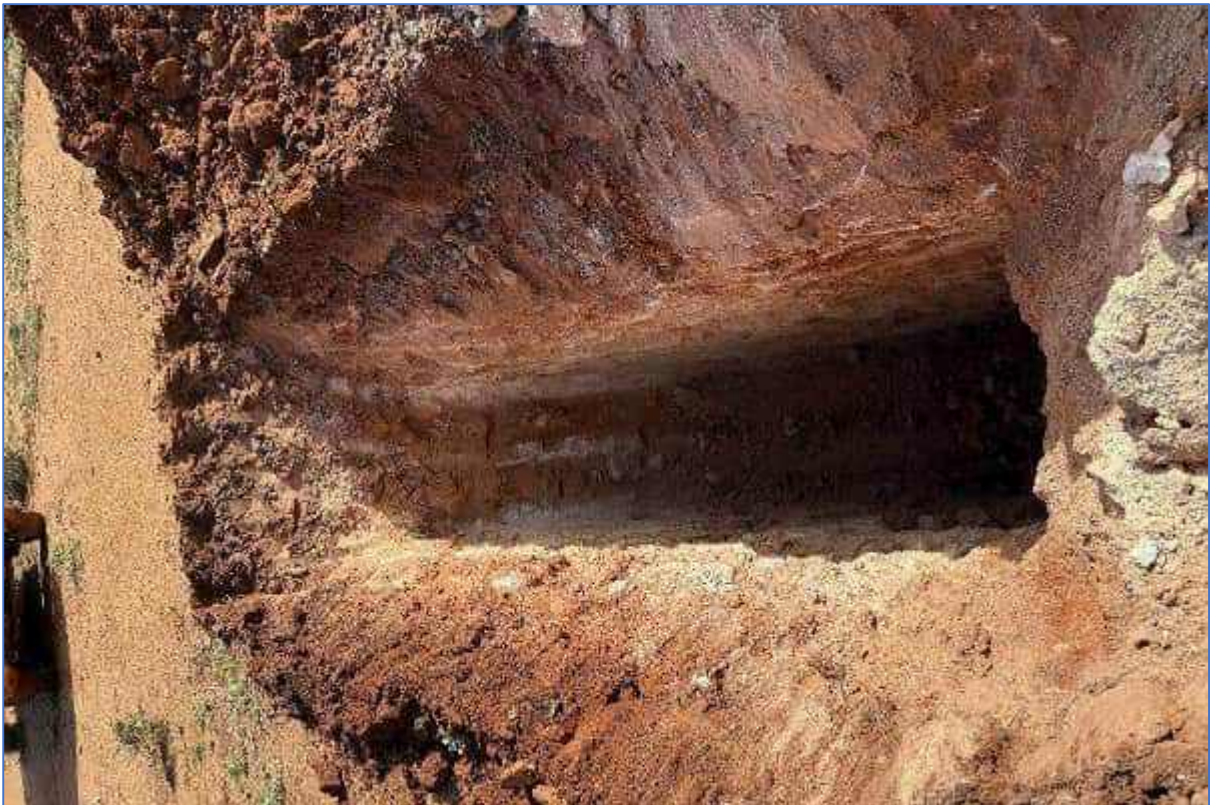
Plate 46: TSF-TP10 – Excavation to refusal
