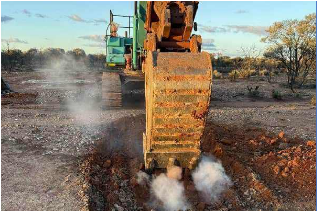
Plate 95: TSF-TP21 – Test Pit location
