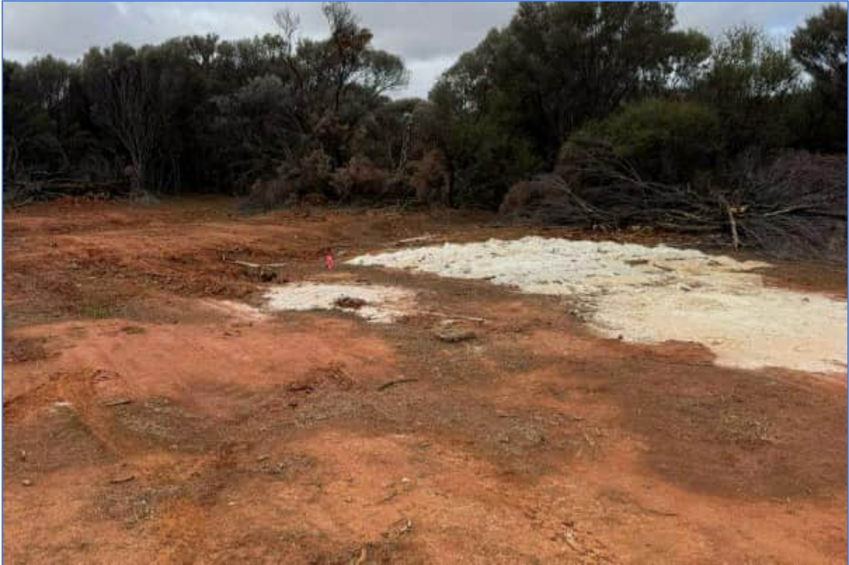
Plate 23: TSF-TP05 – Test Pit location
