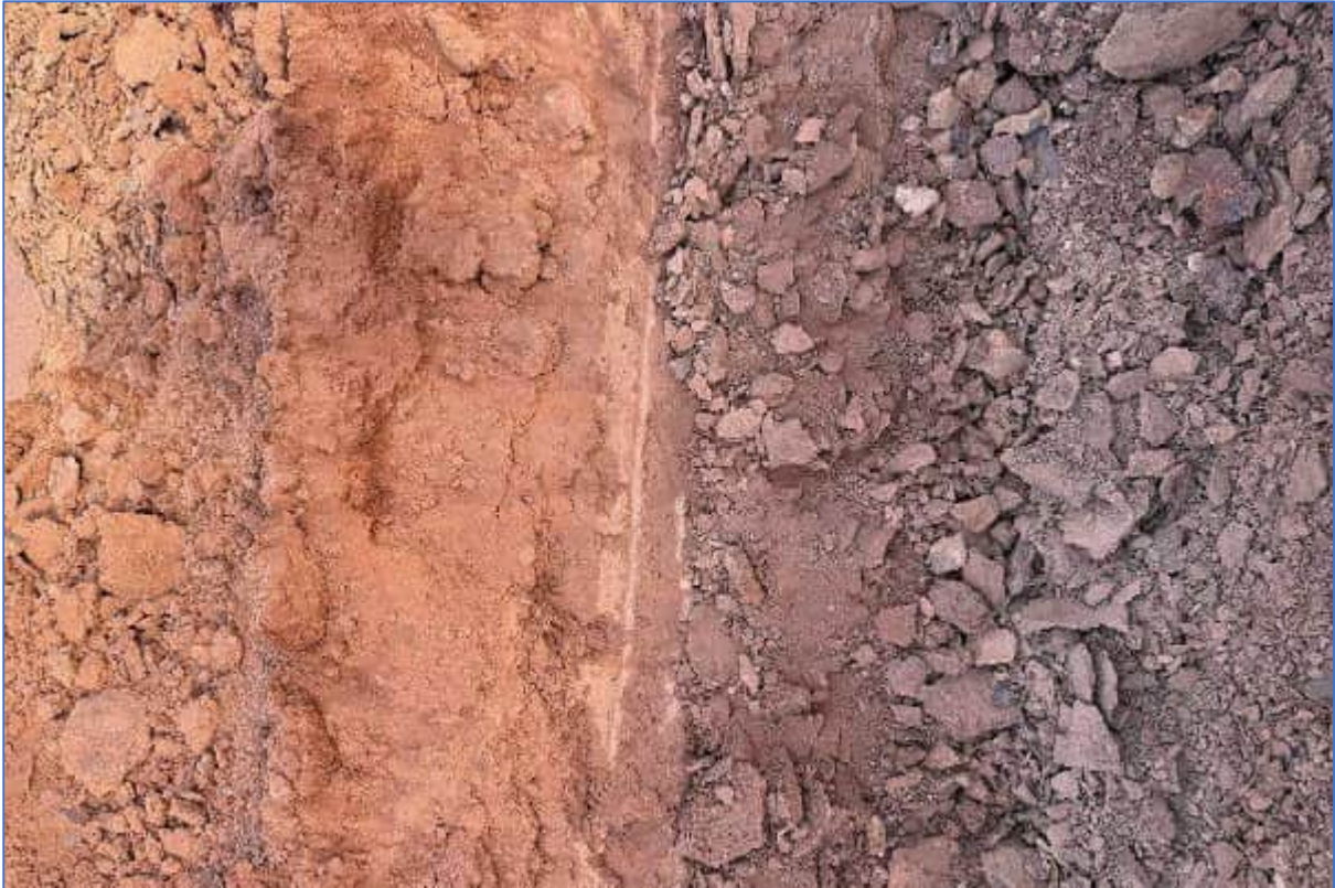
Plate 79: TSF-TP17 – Test Pit wall
