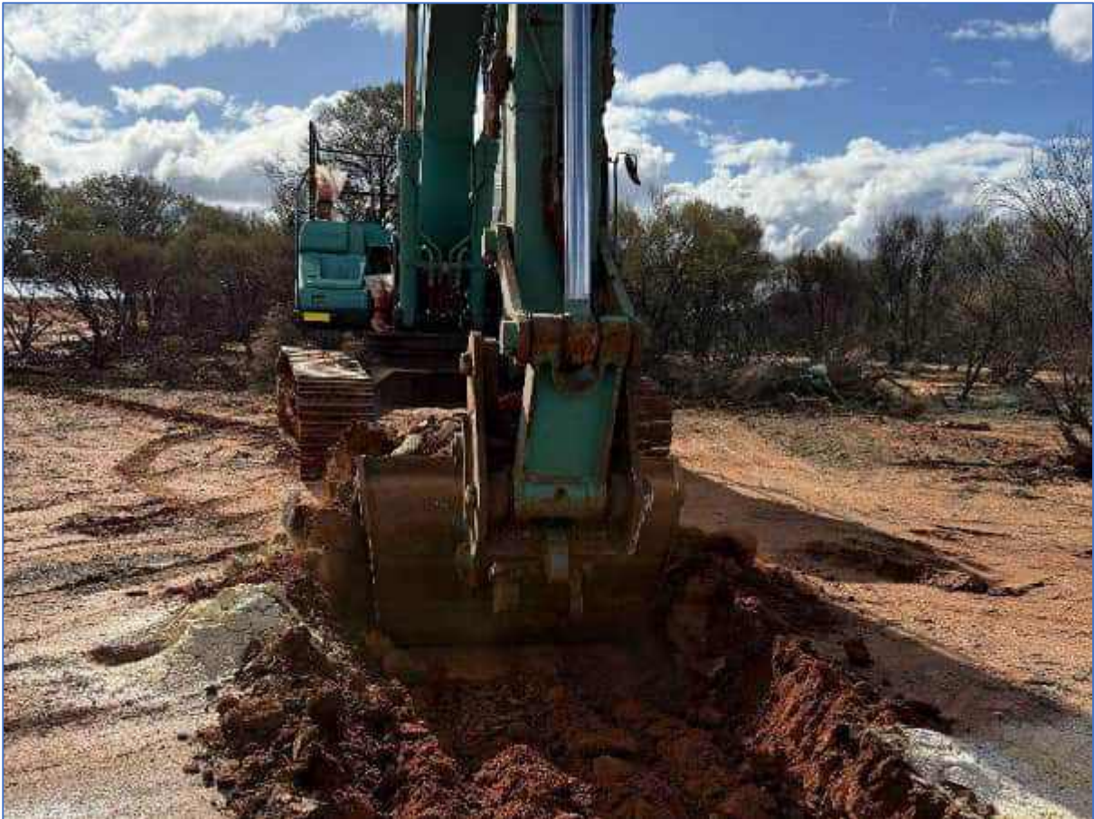
Plate 51: TSF-TP11 – Test Pit location
