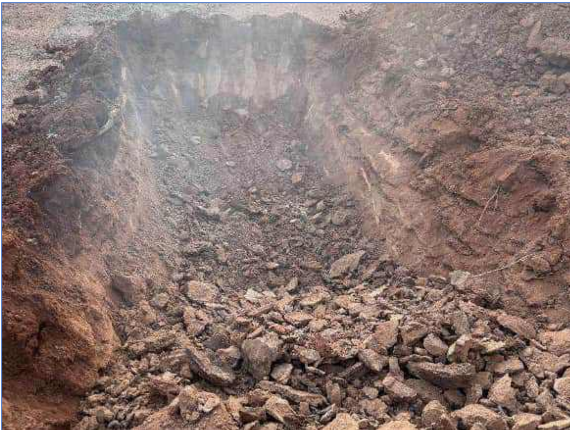
Plate 92: TSF-TP20 – Excavation to refusal
