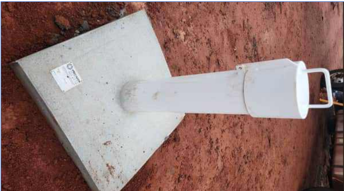
Plate 20: TSF-BH-03 Standpipe Installation
