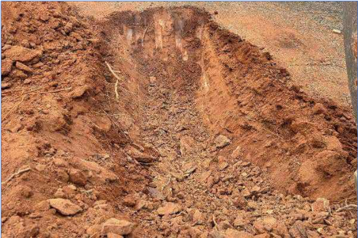
Plate 18: TSF-TP04 – Excavation to refusal
