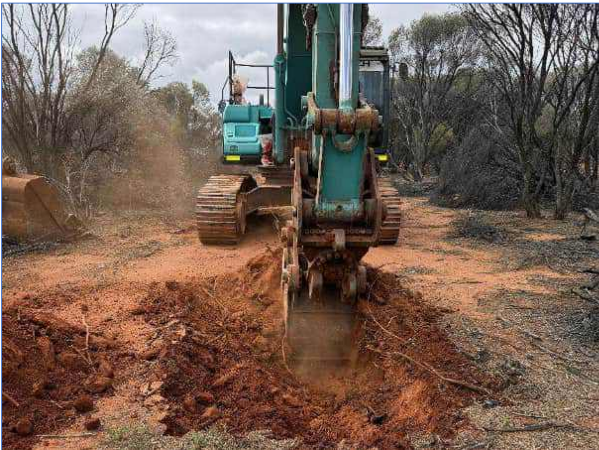
Plate 36: TSF-TP08 – Test Pit location
