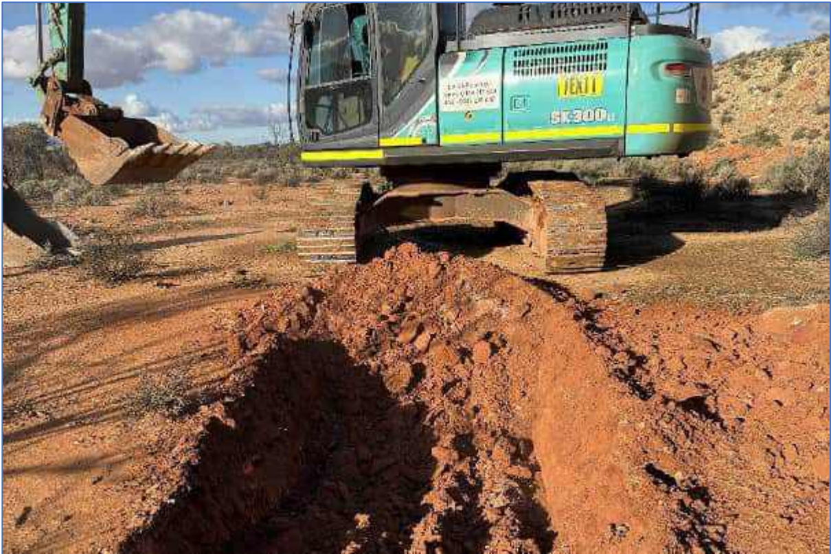
Plate 73: TSF-TP16 – Test Pit location
