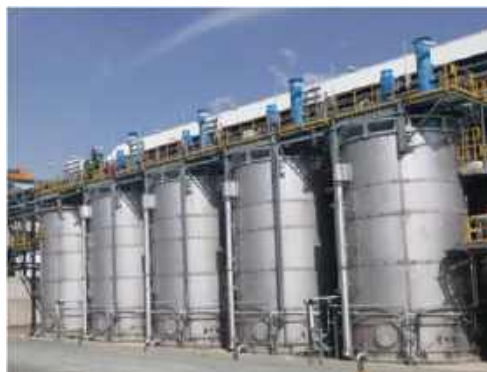
Figure 5-4 – Oxidative Leach Train
