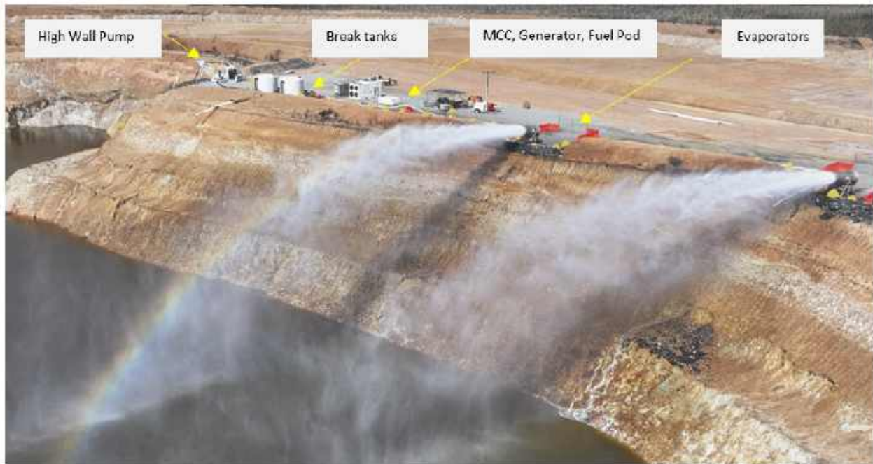
Figure 3: EGGP Evaporator Layout as per W6919/2024/1.
