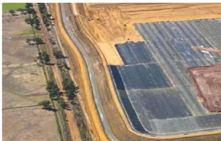
Figure 7-4: Contouring external residue embankment trial.
