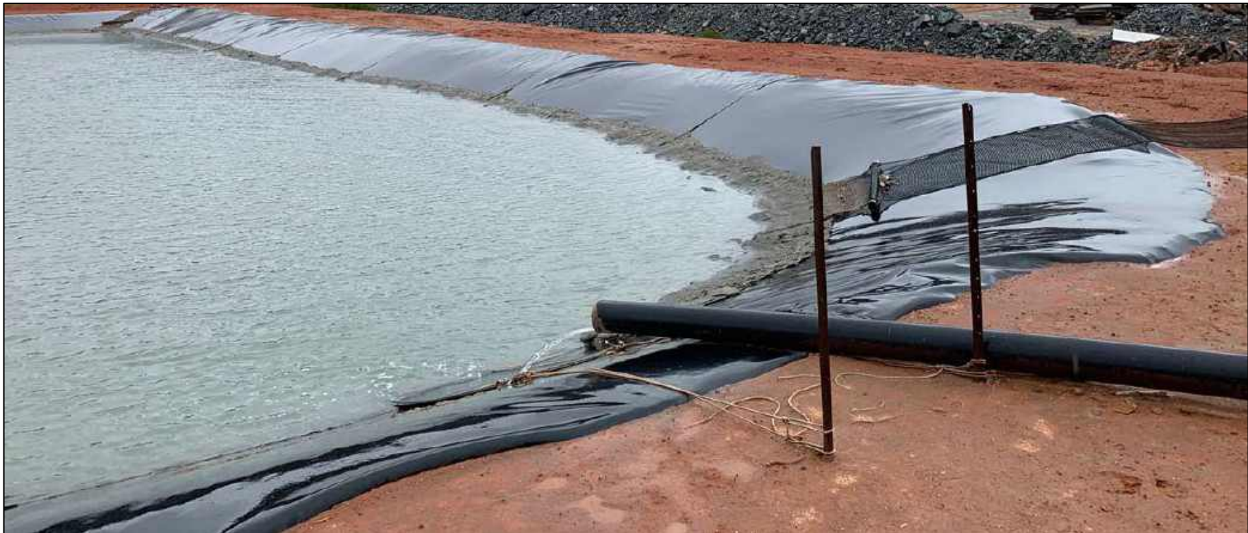
Figure 4: Typical mine water pond
