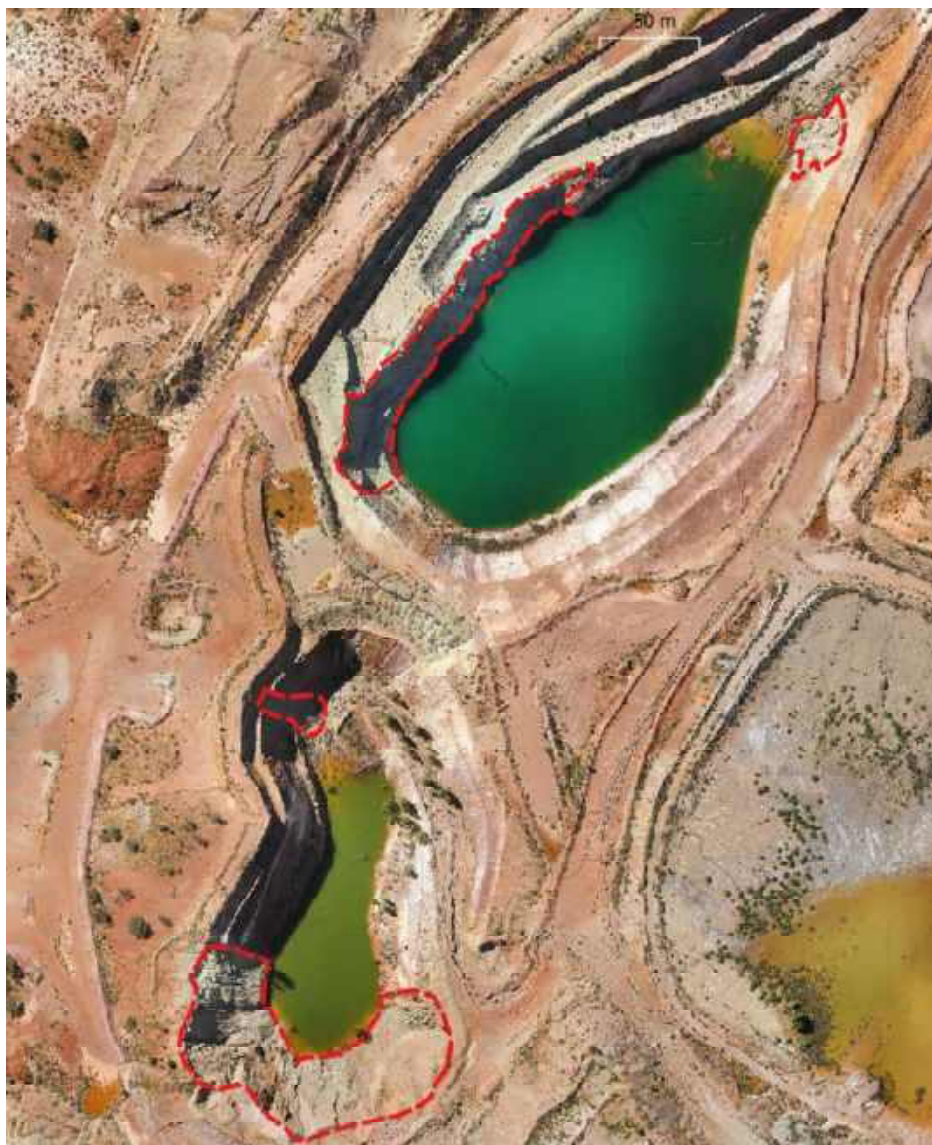
Figure 7.14 Localised areas of pit instability
