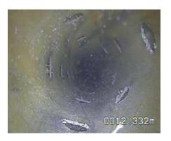
Holes in bore casing water entry into bore
