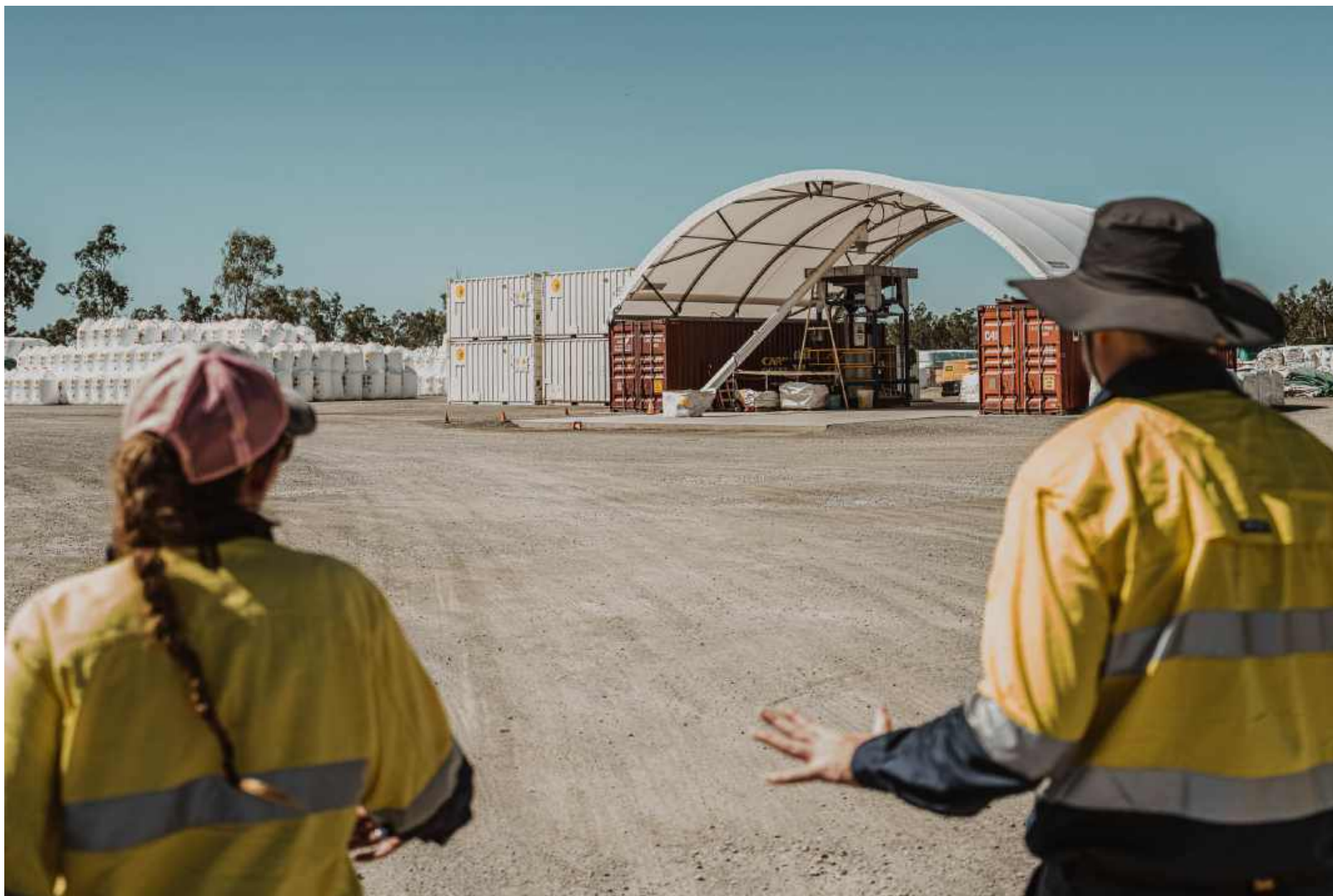
Figure 5 AN loading station where AN is augered into shipping containers for transport to mine sites. This type of loading station will be located between the two dome shelter storage areas.
