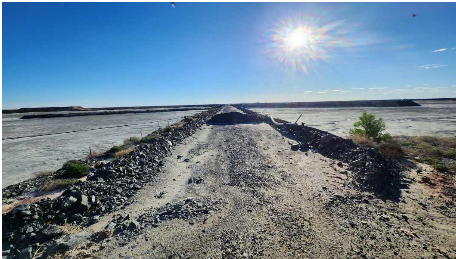
Figure A.14 – Photograph A14: Dividing wall between TSF1 (North) and TSF2 (South)
