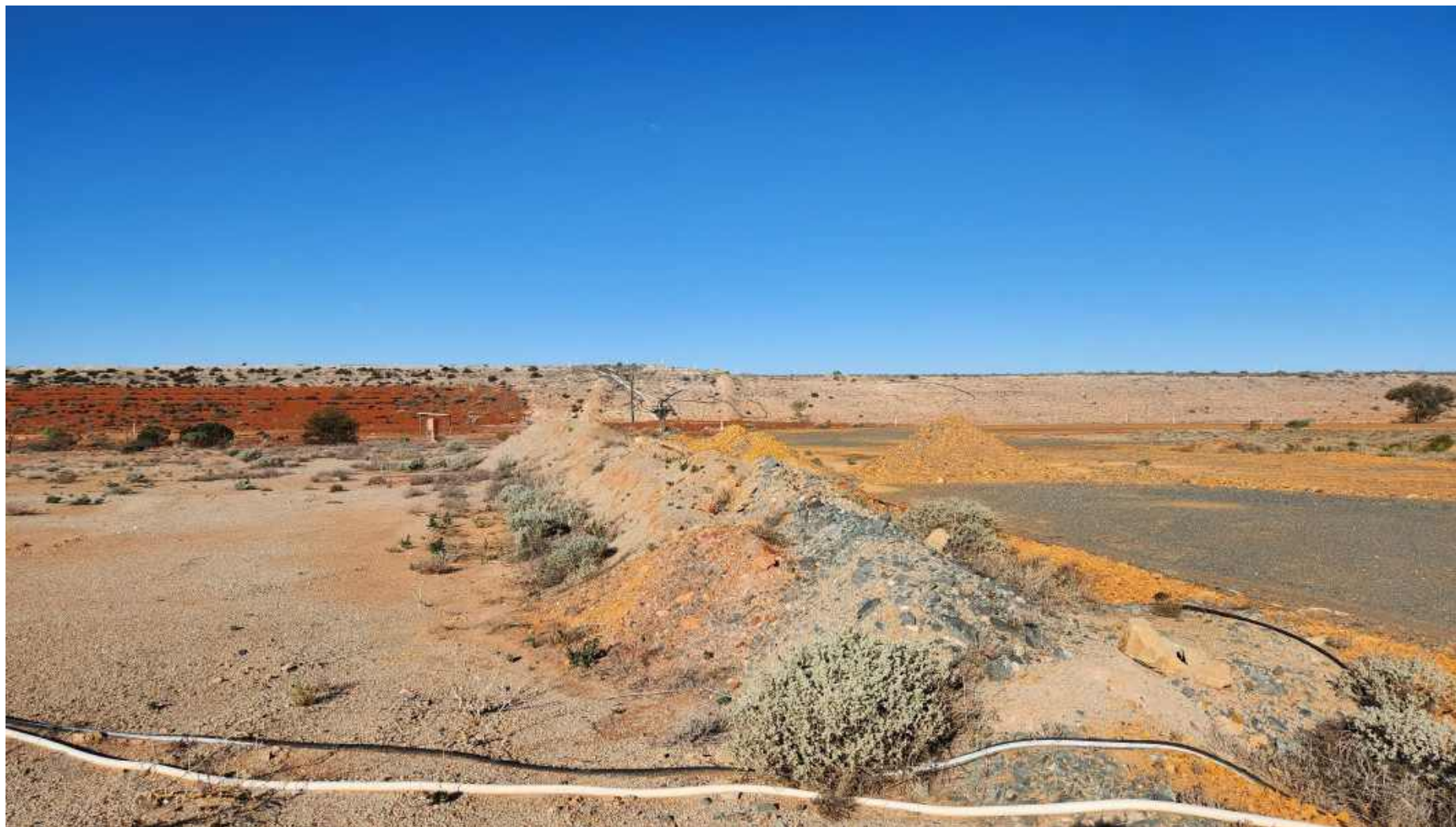
Figure A.9 – Photograph A9: Pipelines leading to TSF1-TSF2 dividing wall
