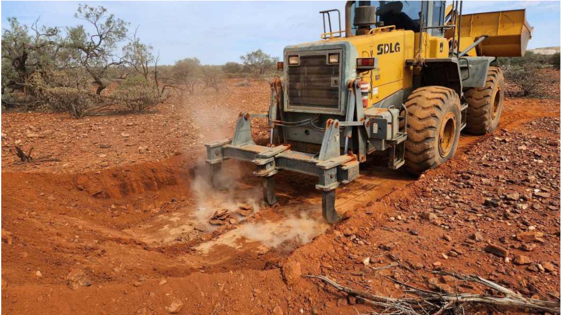
Figure A.25 – Photograph A25: TP10 (ripper refusal)
