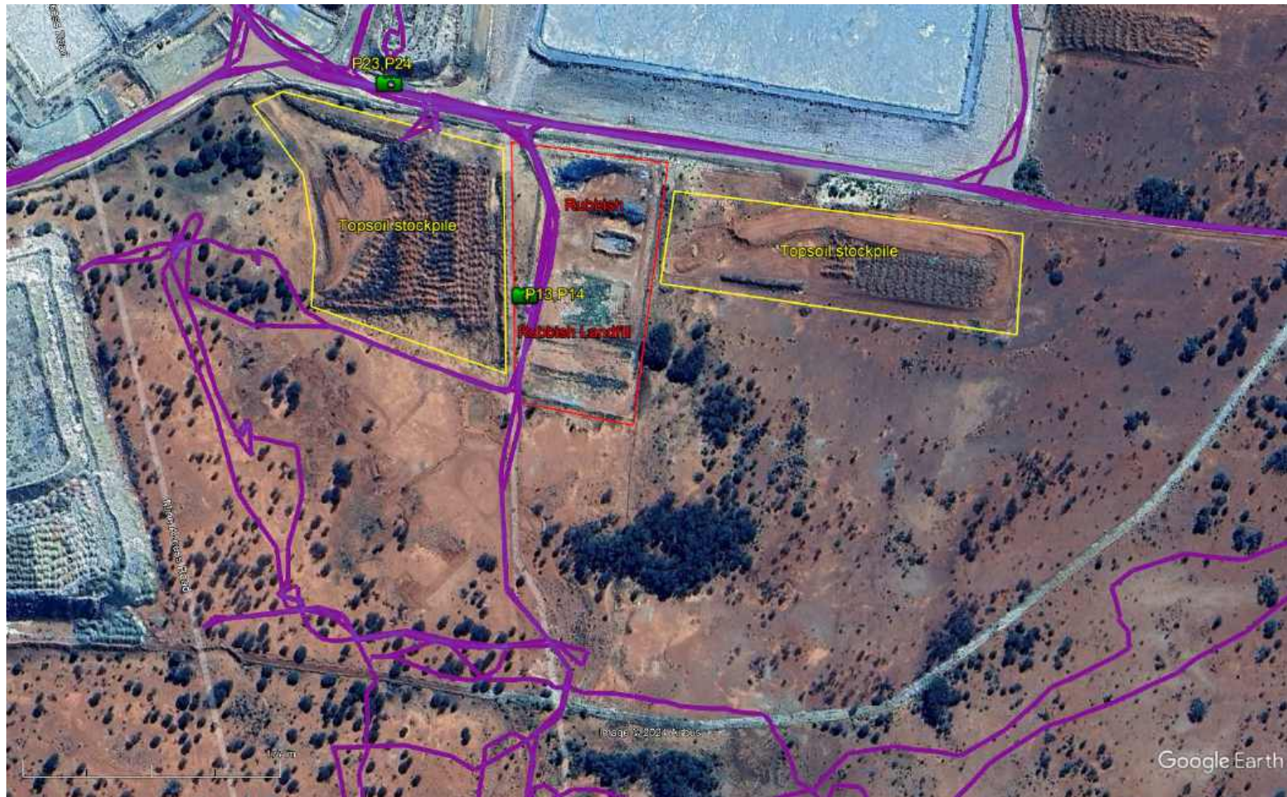
Figure 4.3 - Presence of topsoil stockpile, exposed rubbish stockpile, and putrescible landfill area
