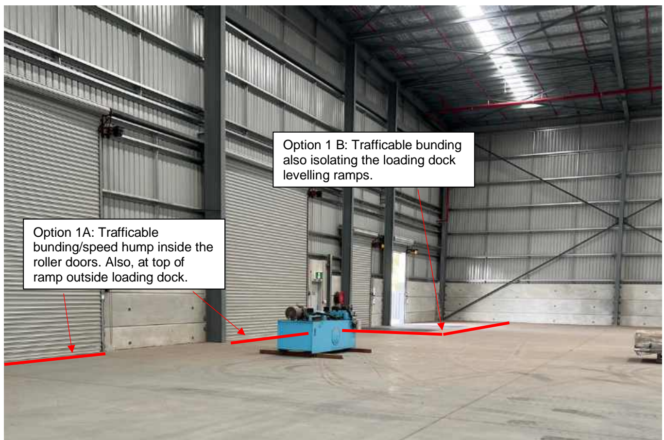
Figure 5 Fire water containment options at roller doors and loading dock levelling ramps
