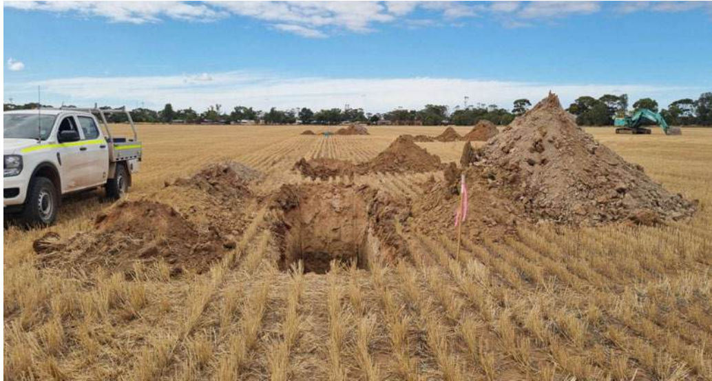
Photograph 3: Test pitting at TP01
