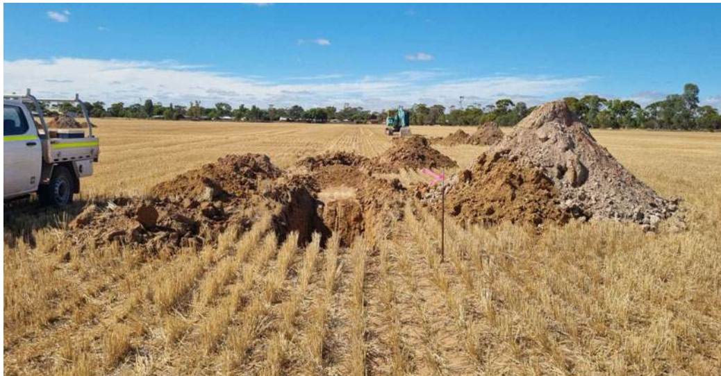
Photograph 4: Test pitting at TP05
