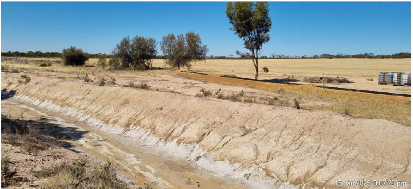
Photograph 5: Table drain about 700 m east of site traversing north south, note erosion gullies
