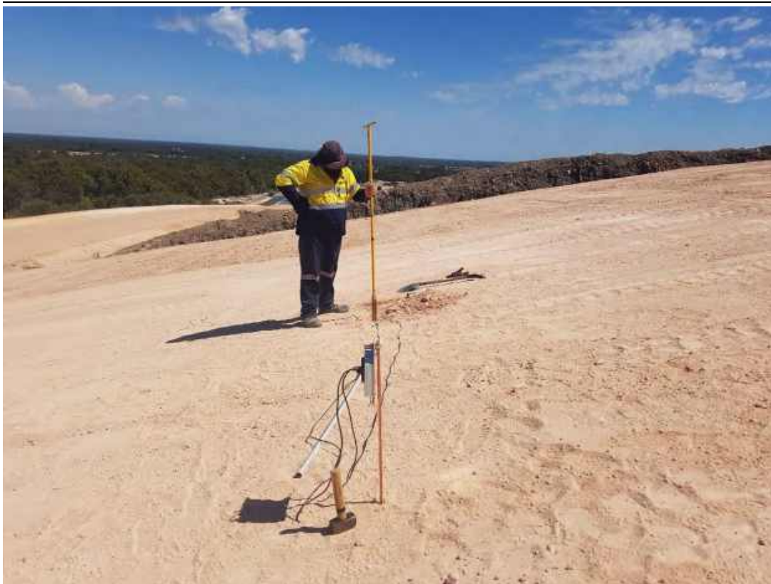
Plate 6 Sensors installed using a narrow hand auger after excavating a shallow trench
