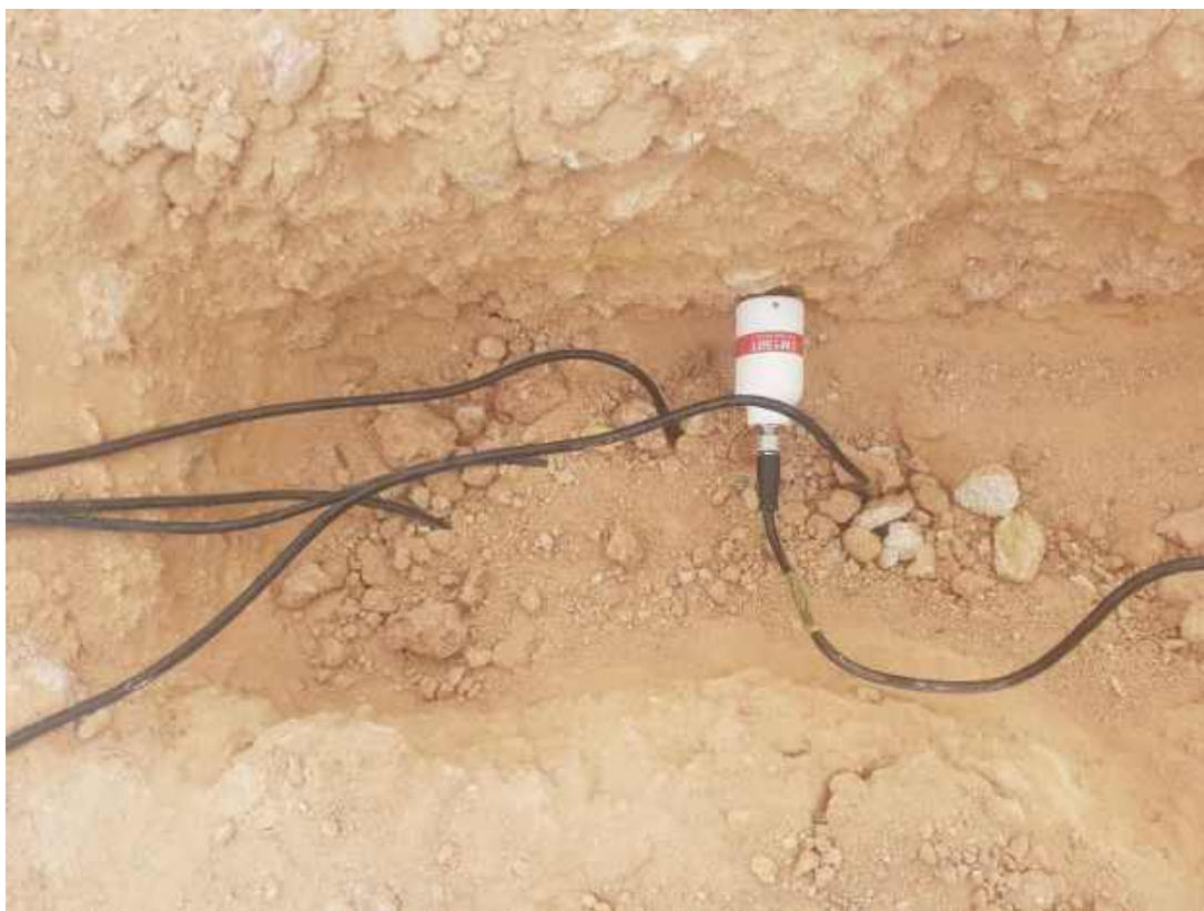
Plate 7 Shallow trench showing backfilled deeper sensors (installed vertically) and the shallow sensor at 20 cm installed horizontally in trench wall
