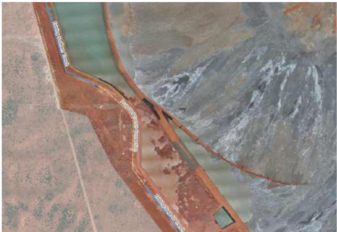
Figure 7: Proposed Linkage of the Southern Seepage Interception Trench with the Stage 10 Seepage Interception Trench
