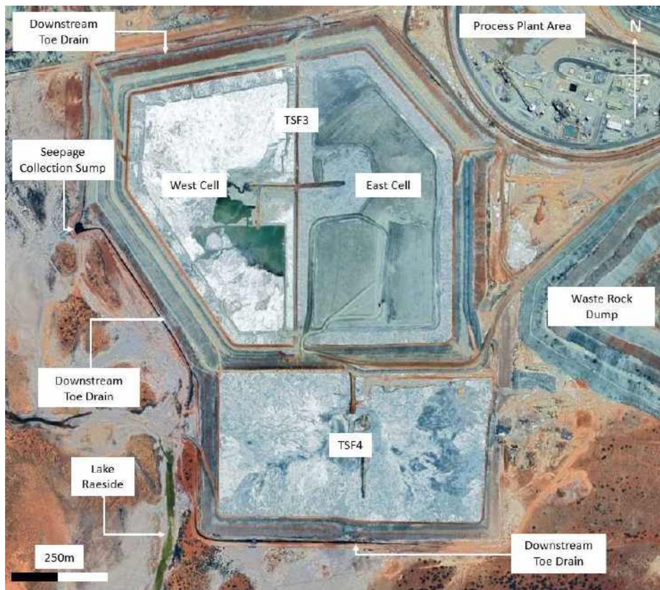
Figure 1.1 Overview of the Gwalia Gold Mine TSF3 and TSF4 (image from Google Earth, 2023)
