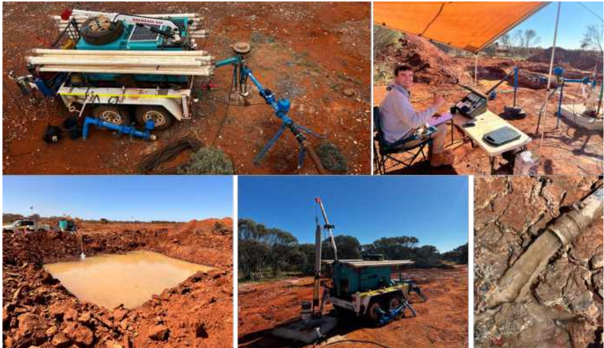
Figure 3-2 Pump testing of the depressurisation / seepage recovery bores.
