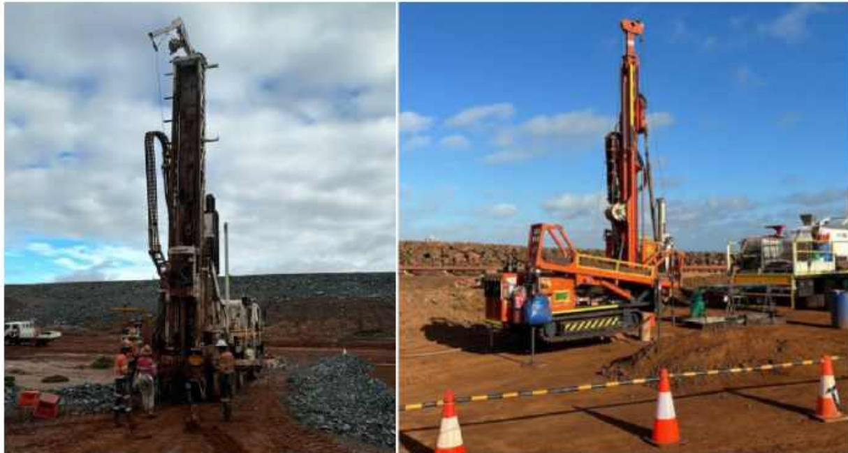
Figure 3-1 Seepage / depressurisation drilling at the Project (Left) and the piezometer drilling using the Hanjin D8 rig at the project (Right).
