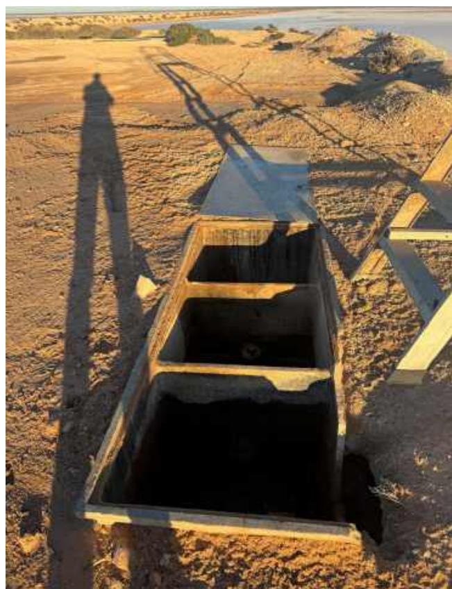
Figure 9 - SW18 Triple Interceptor
