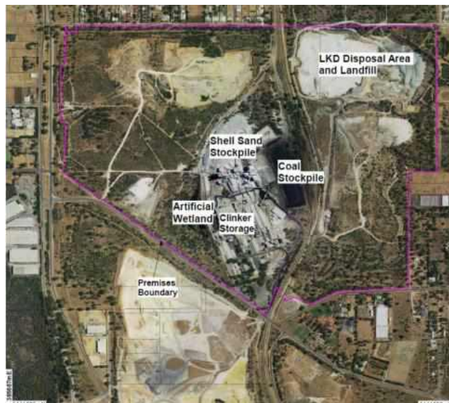
Figure 1: LKD Disposal Area and Landfill
