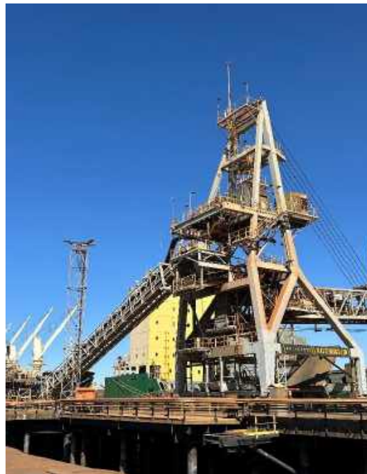
Figure 3: Shiploader on Berth 1 at the Premises (L4432)
