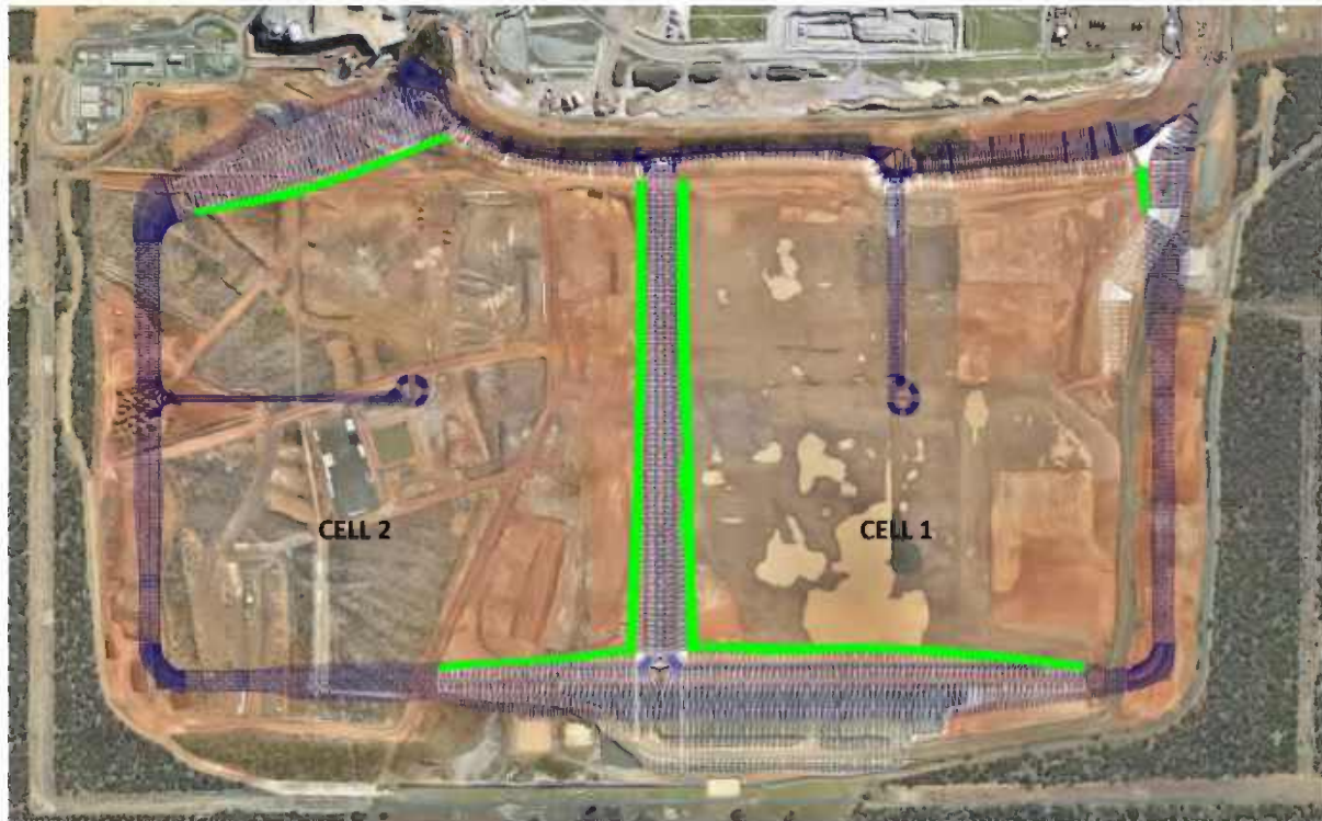
Figure 21: Cell 1 and 2 1,270mRL embankment raise
